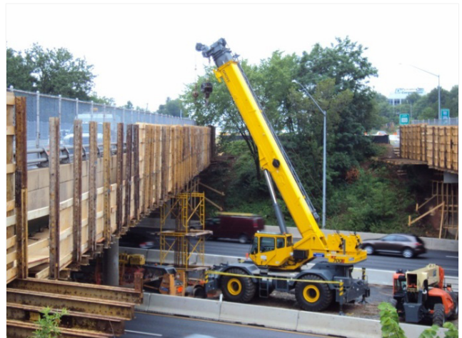
Figure 5-2. Example of Bridge over Roadway with a Crane
