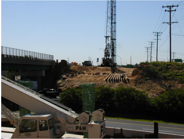
Figure 5-1. Example of Pile Driving Equipment
