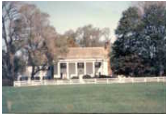
View from field in front of house
