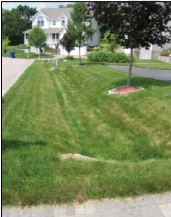
Figure 2: Example of Grass Swale
