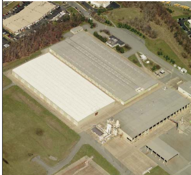
Existing development in the I-2 zone
