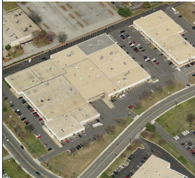
Existing development in the I-1 zone
