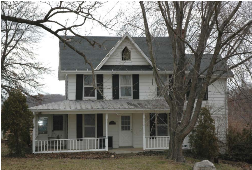
15/4 Alfred Baker House, 28901 Kemptown Road
