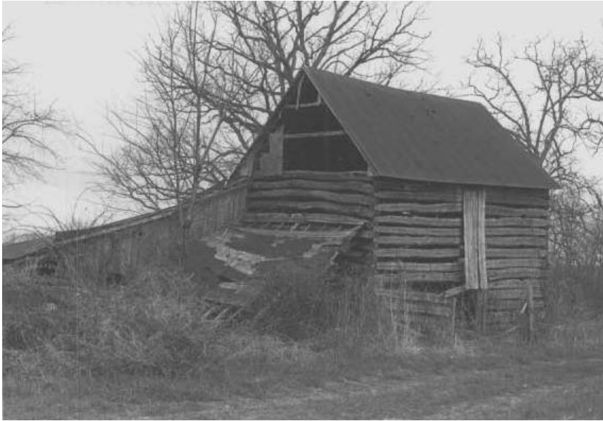
Barn on original Halterman Road site, 1979 view
