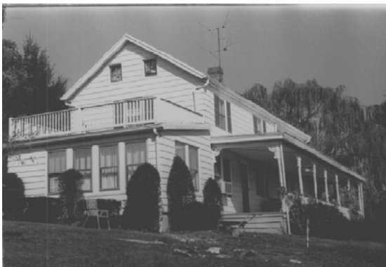
Log House, no longer standing
