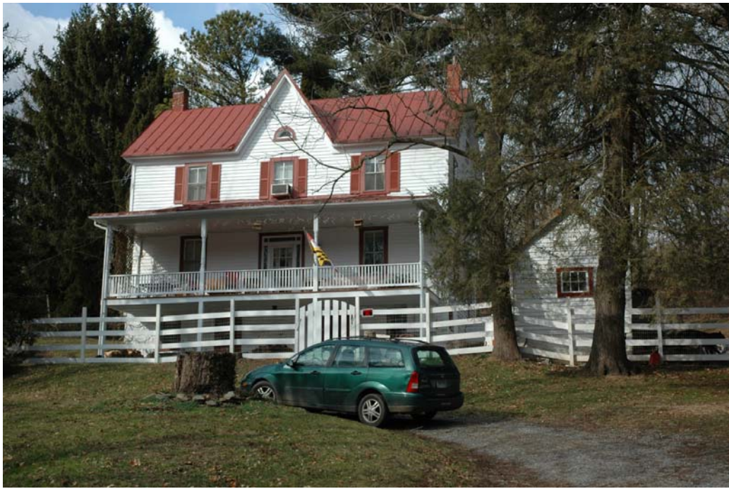
15/71 Chrobot House (Margaret Price House), 24724 Hipsley Mill Road Not Currently Listed on the Locational Atlas and Index of Historic Sites
