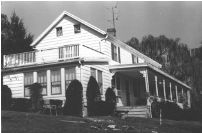
Log house, no longer standing
