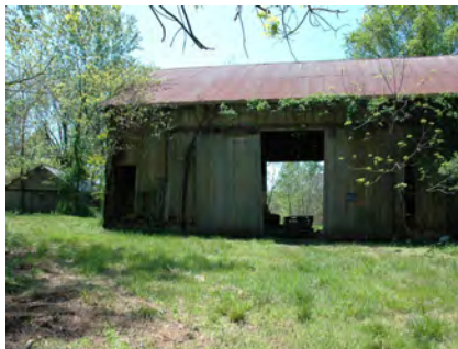
Barrack barn, Site 1
