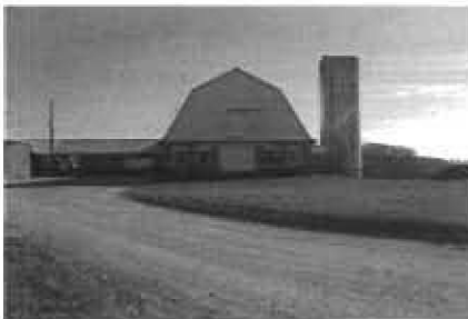
Dairybarn and silo
