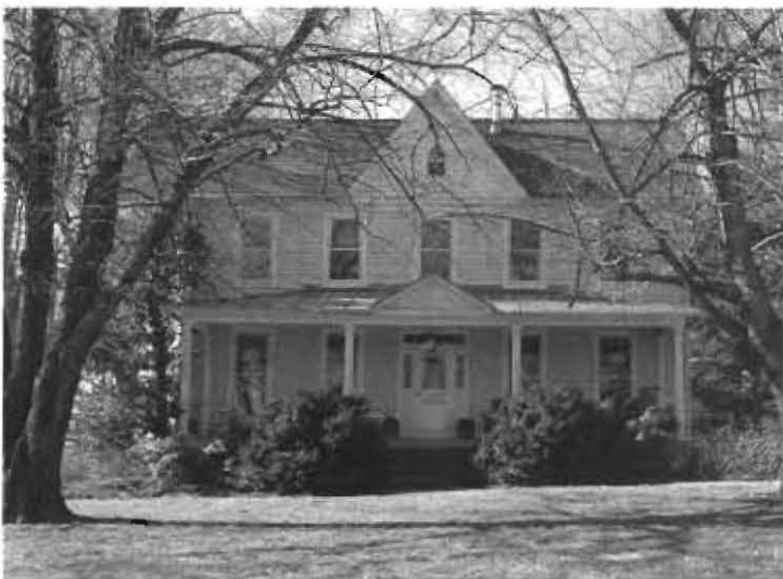
15/5 Molesworth-Burdette House, 28600 Ridge Road, front facade
