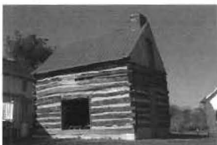
Tobacco house, demolished October 2010
