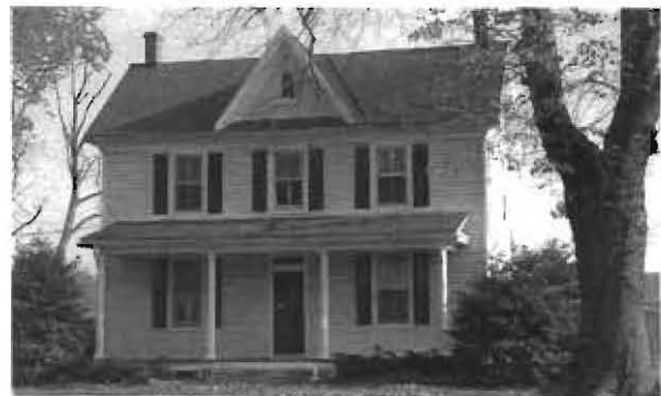
15/29 Etchison Historic District, William and Pearl Moore House, three bays wide, 24221 Laytonsville Road
