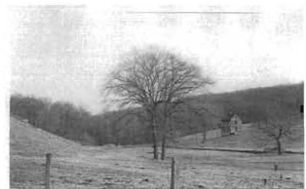
Tenant House, Shibley-Mullinix Farm (15/13), c1970 (Mike Dwyer)
