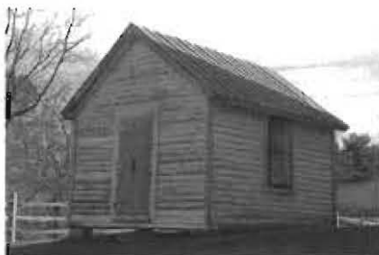
Domestic outbuilding, demolished October 2010
