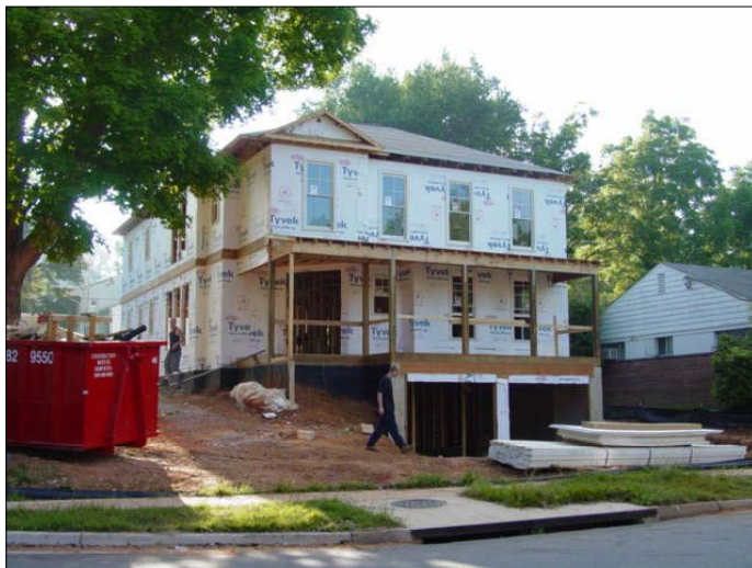
A large house under construction towers over its neighbor, but is built according to code. Such disparities in height prompted citizens to lobby the County Council for zoning revisions.
