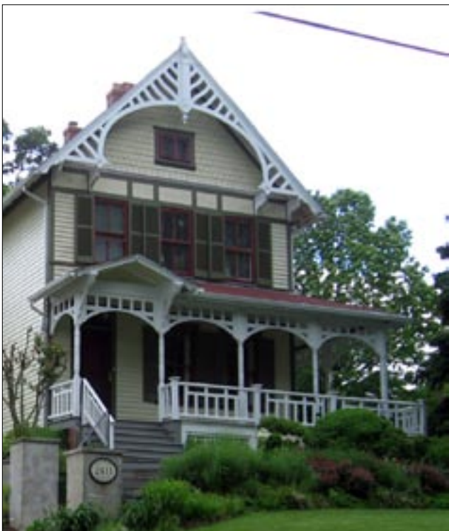
Guideline 1.1: The wrap around front porch, uniquely designed balustrade, post brackets, and ornate barge board are all character-defining features of this structure that should be preserved.
