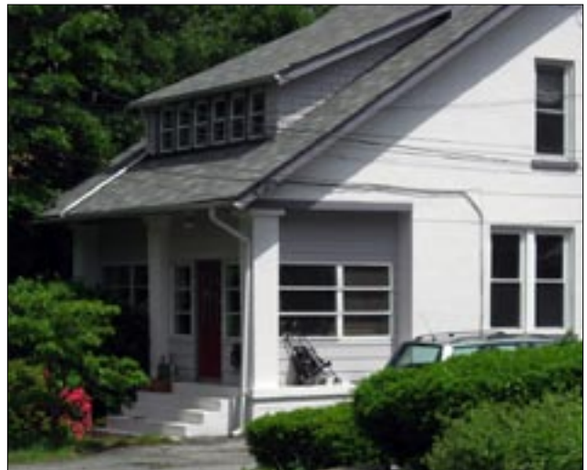
Guideline 3.4: Consider restoring an altered porch back to its original design and configuration. In this case, the enclosed porch would once again be open.
