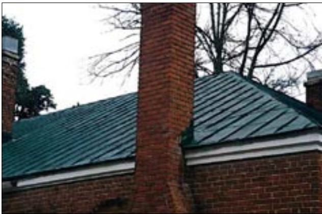
A metal seam roof is a traditional roof material and should be preserved and maintained.
