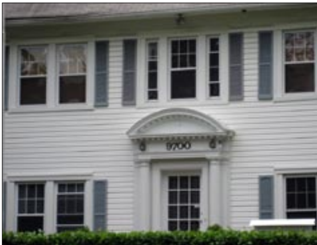
Guideline 4.3: Maintain the historic window arrangement including the flanking shutters.
