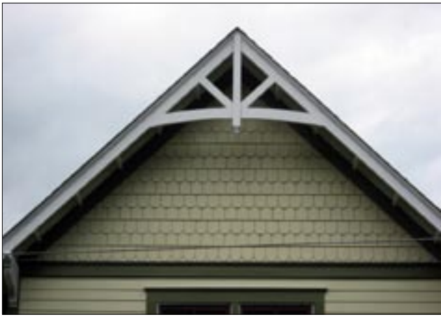
Guideline 5.3: Preserve the original eave depth of a historic roof.
