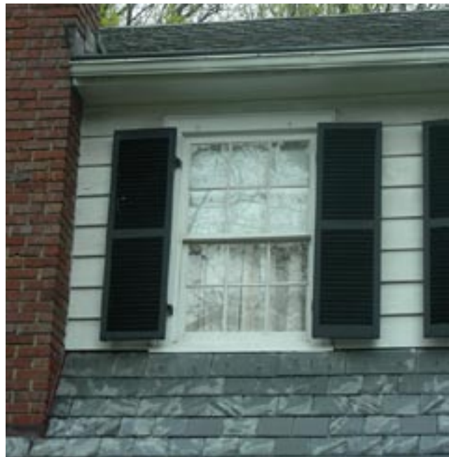
Slate is a traditional material used on roofs in Montgomery County.
