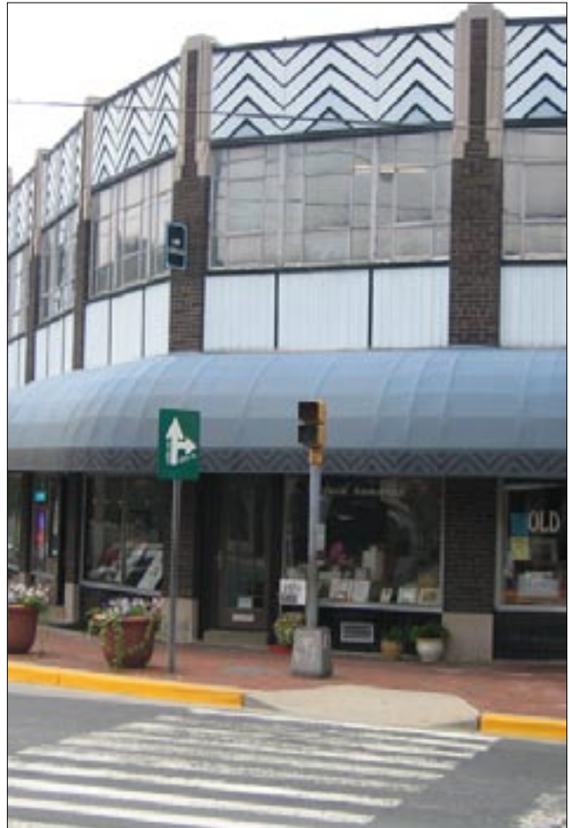
Art Deco storefronts are seen throughout Montgomery County. This storefront includes large display windows and kickplates.
