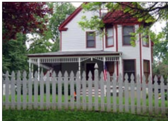
Guideline 12.2: A fence that defines a front or side yard on a corner should be low to the ground and transparent in nature.
