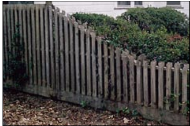
Guideline 12.4: Consider a gradual increase in fence height from the front side yard to rear side yard.
