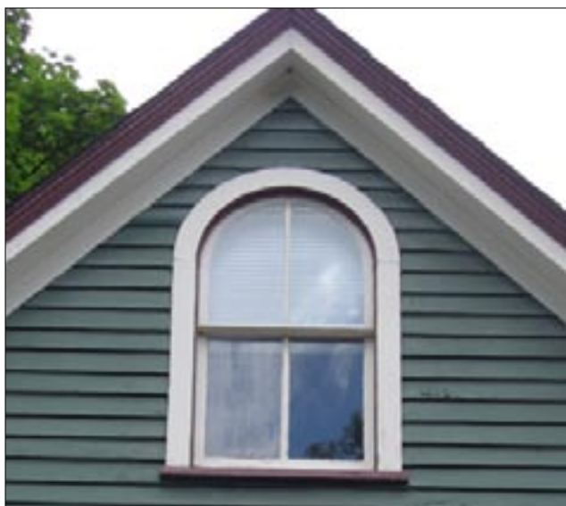
Muntins on historic structures are typically wood.
