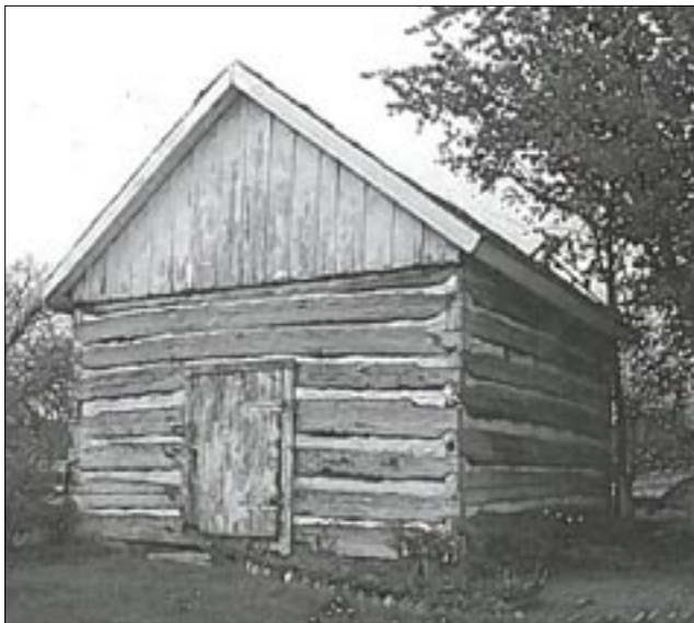
Smokehouses typically have a gabled roof form and simple rectangular building plan. (Rocklands Farm)
