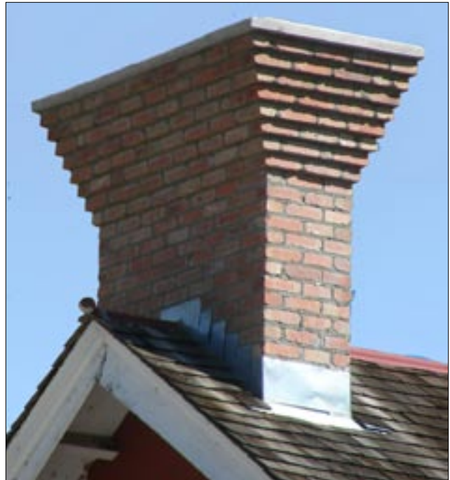
Guideline 6.1: Retain the original height, details, profile and materials of the chimney.
