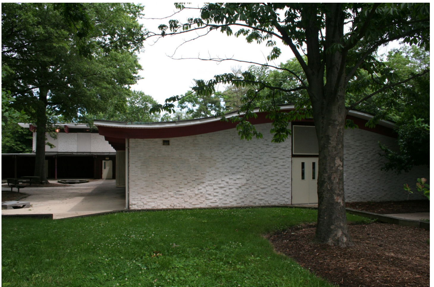
FIGURE 10: South Elevation. (Clare Lise Kelly, June 2013)
