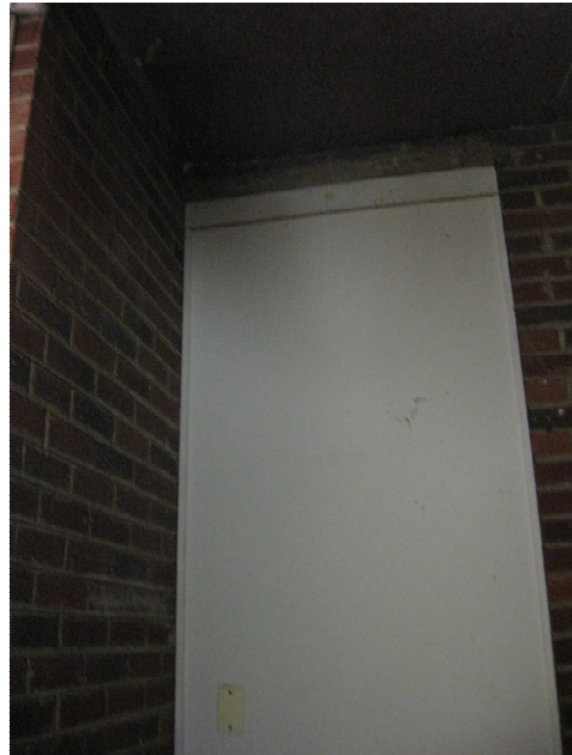
enclosed exterior door to back porch
