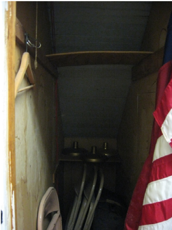
Closet under box stair
