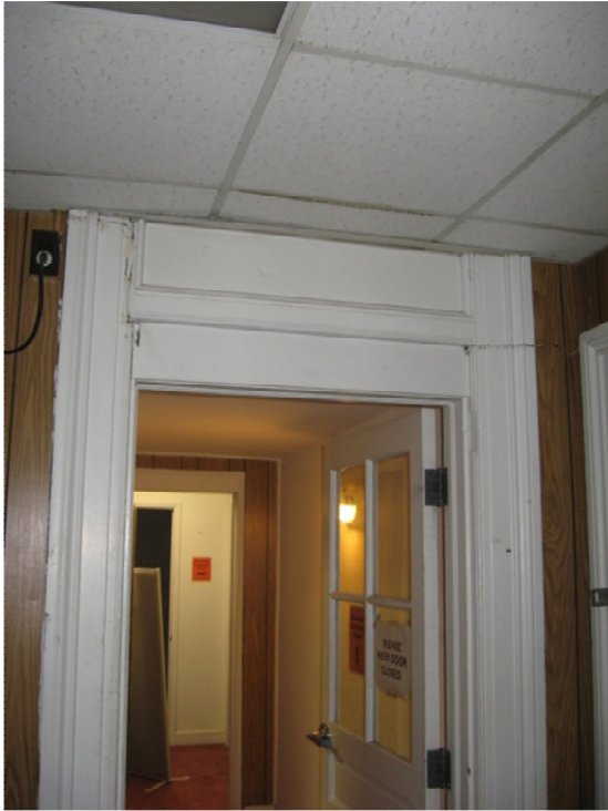
Original doorway into addition
