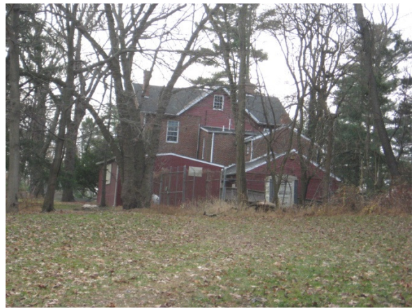
Stubs House rear, north façade
