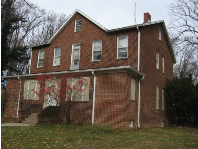
Stubs House front, south façade
