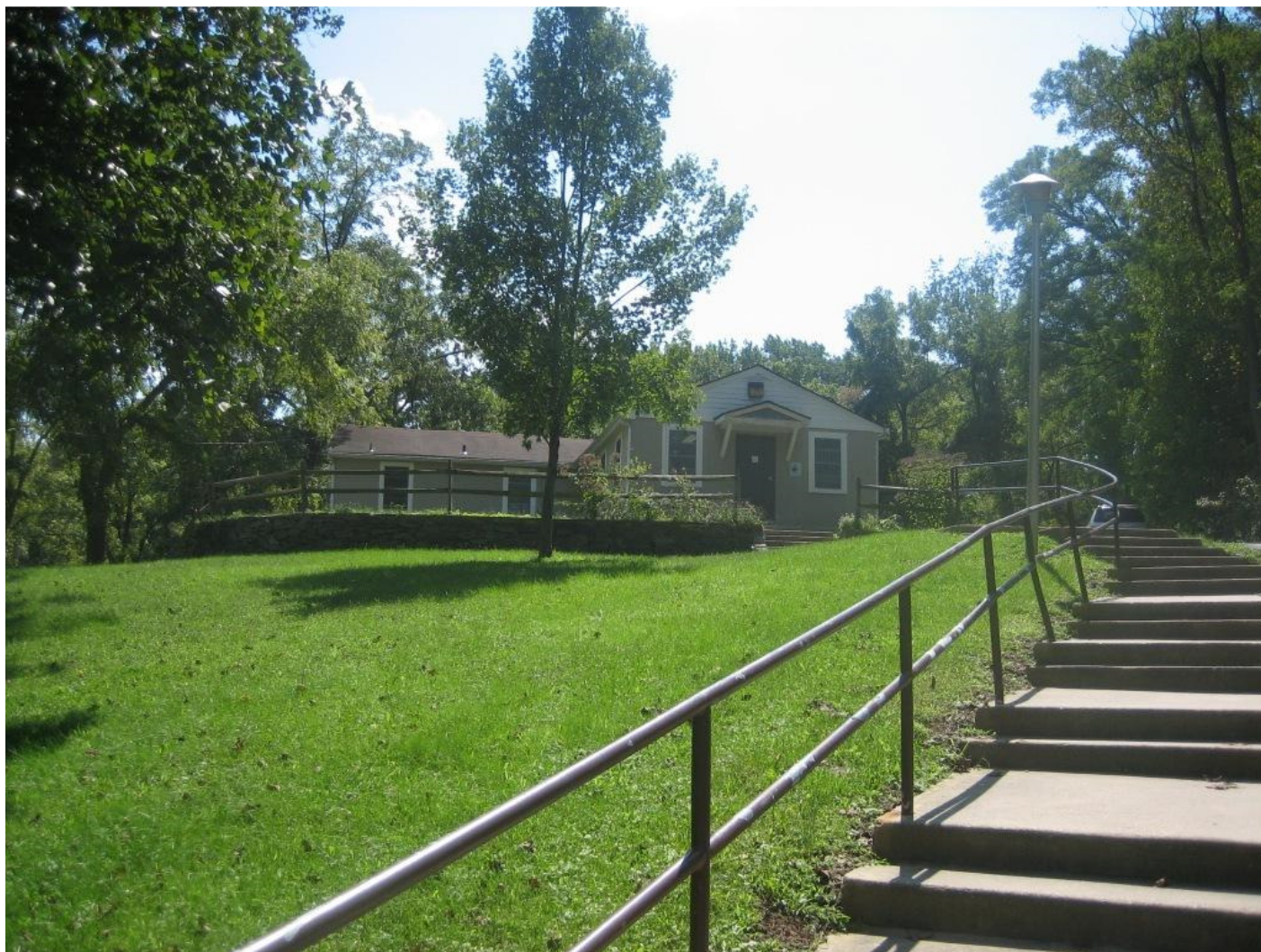
Figure 9. View of Ken-Gar – Palisades Recreation Center, front (north) façade.
