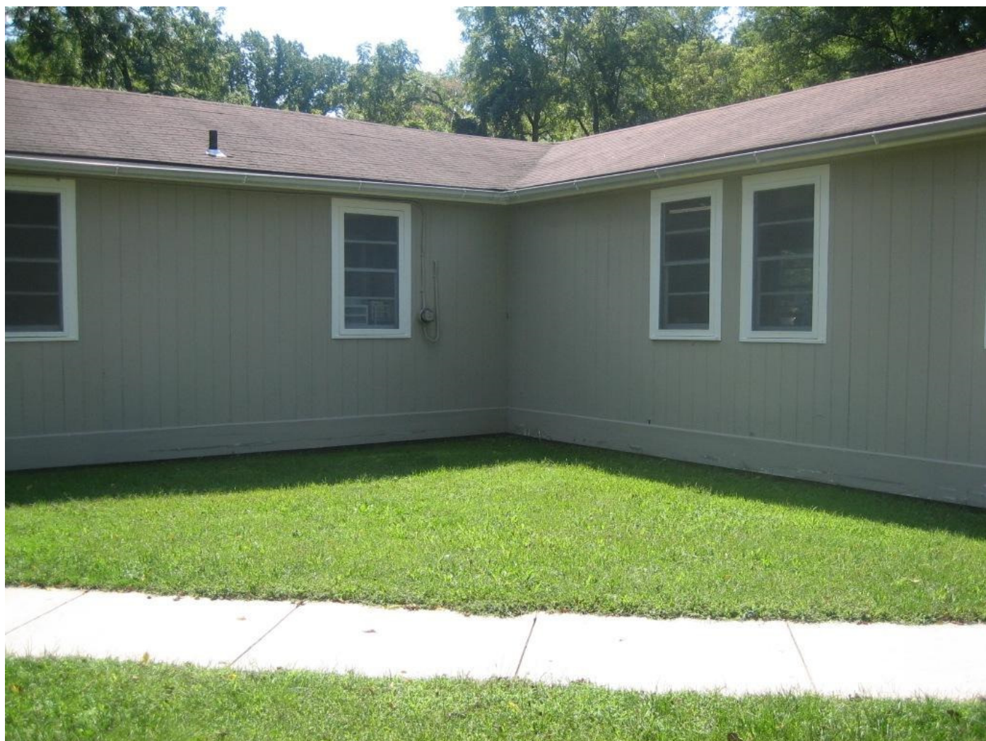
Figure 10. View of Ken-Gar – Palisades Recreation Center, northeast corner.
