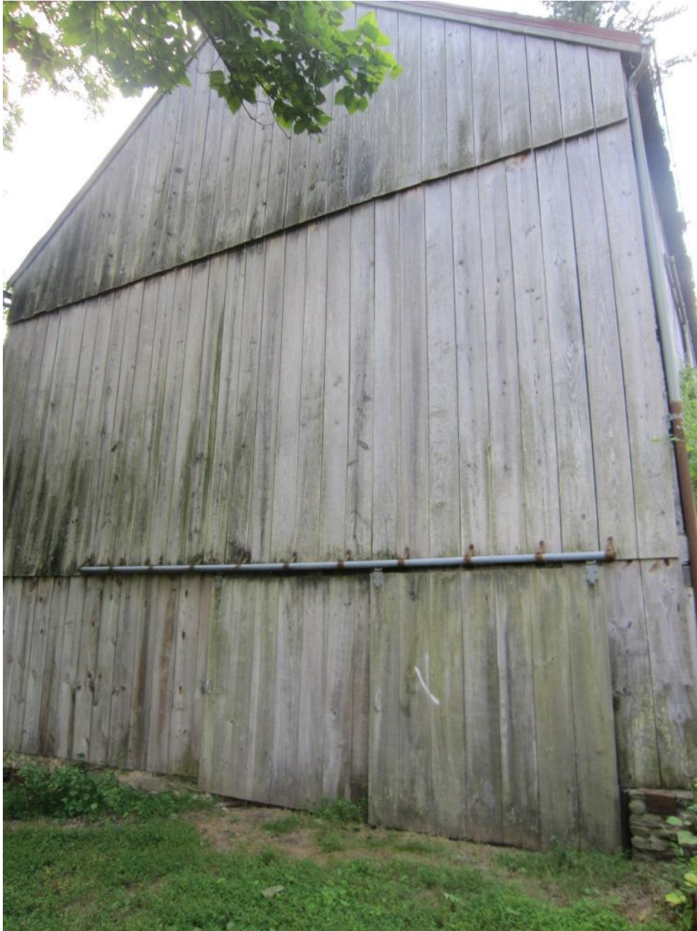
Figure 15. View of the Northeast face.
