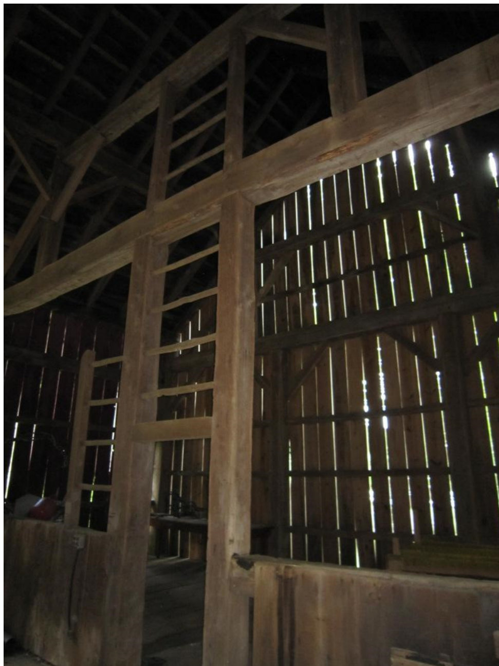
Figure 18. Interior Ladders, Hay Mow Short Walls, Double Tie Beams, and Wall Construction.
