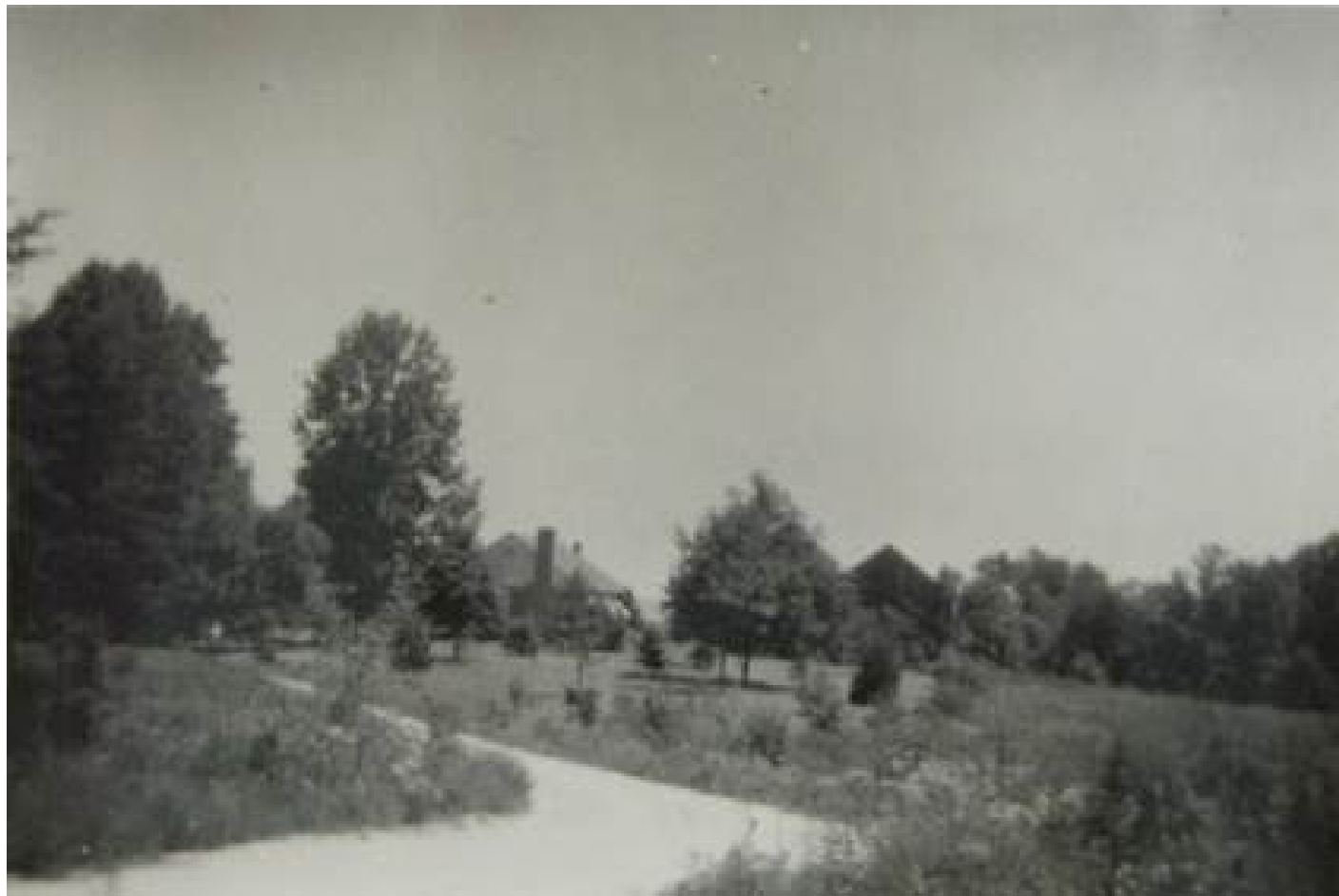
Figure 5. Mid-20 th Century view of the Armstrong property with the Stubbs Barn in the background. Courtesy: M-NCPPC
