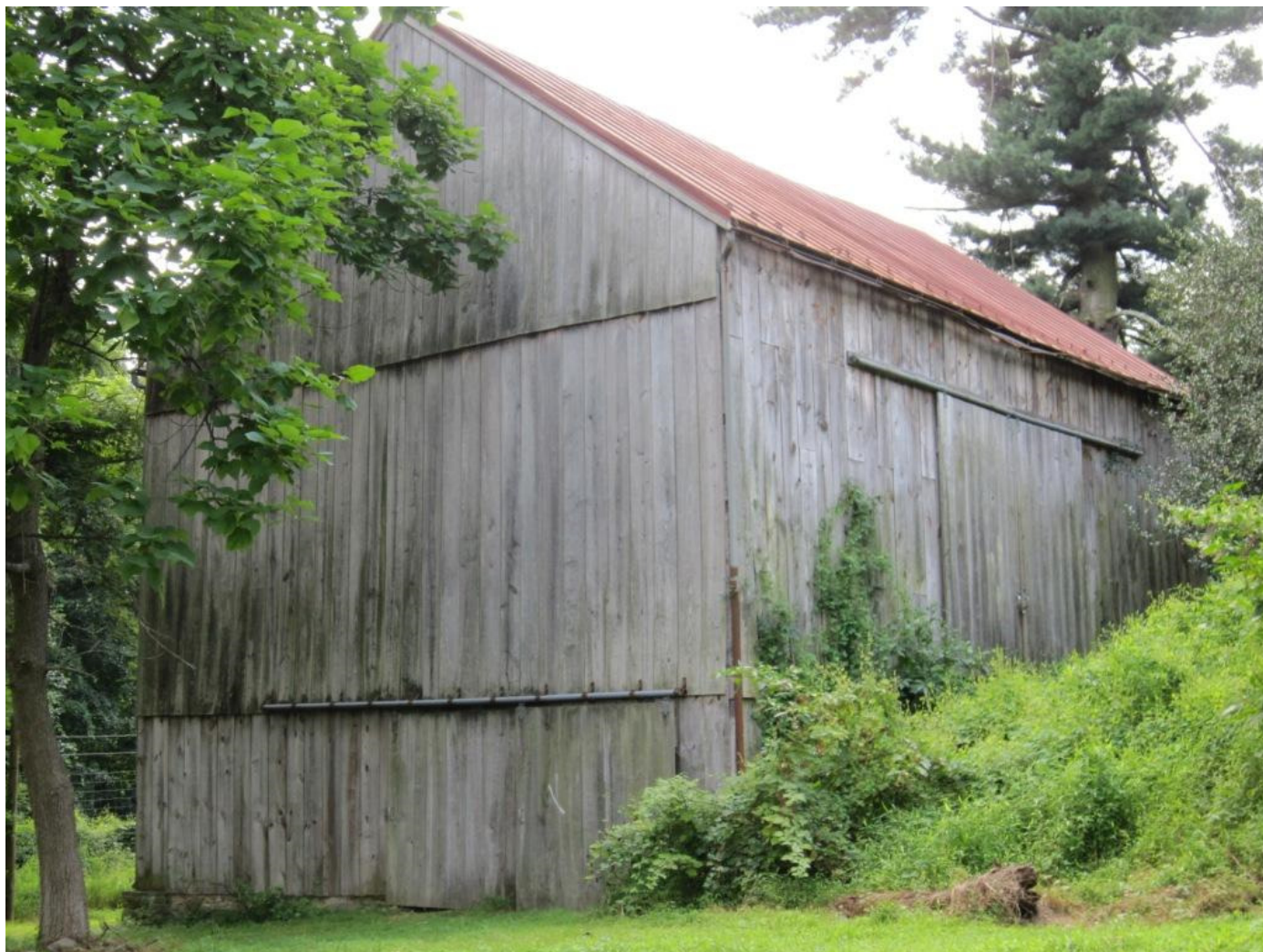
Figure 14. Northwest (front façade) at right, with Northeast gable end.
