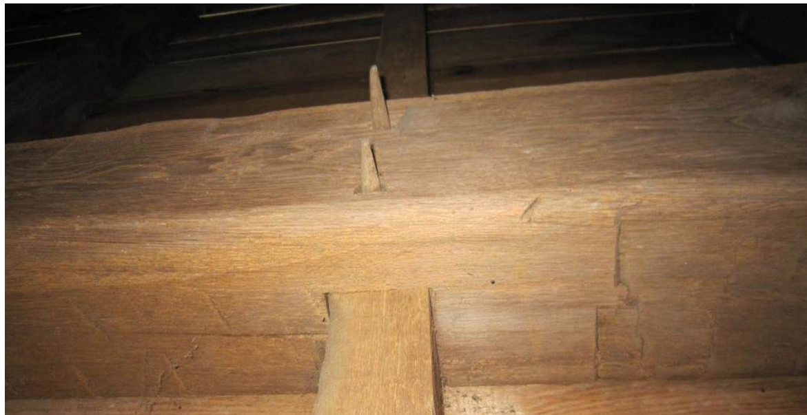
Figure 20. Pointed Pegs between Post and Tie Beam.
