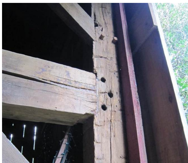
Figure 21. Hewn Interior Post showing missing pegs at Tie Beam.
