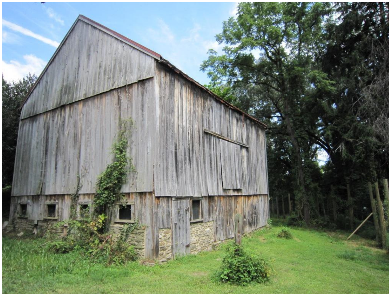
Figure 16. South corner, with Southeast (rear) at right.
