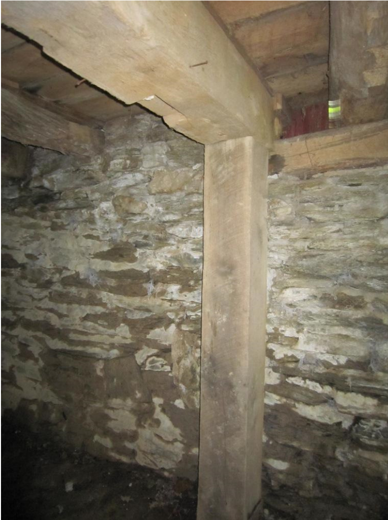
Figure 23. Interior detail, stable level: whitewashed walls and joist framing.
