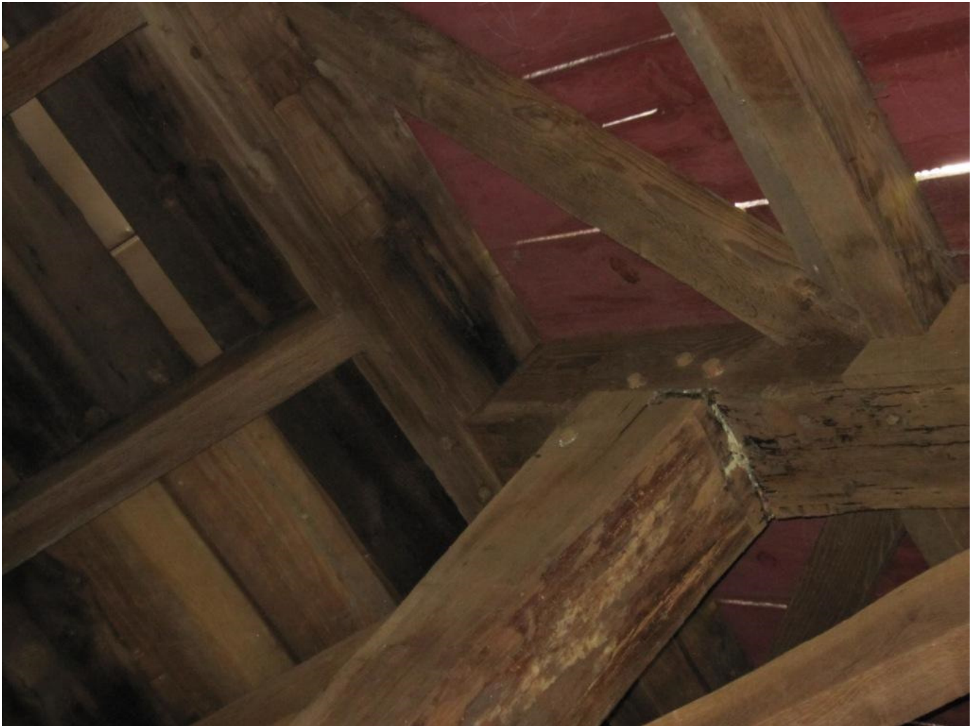
Figure 19. Framing system shows pegs and diagonal braces.
