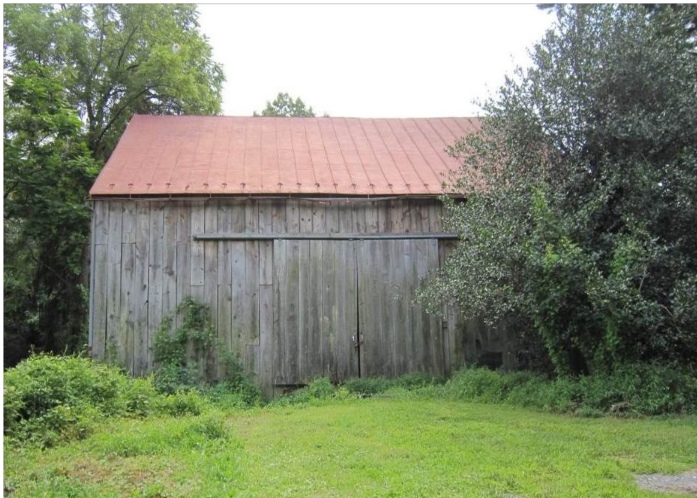
Figure 13. Current view of Northwest front façade.
