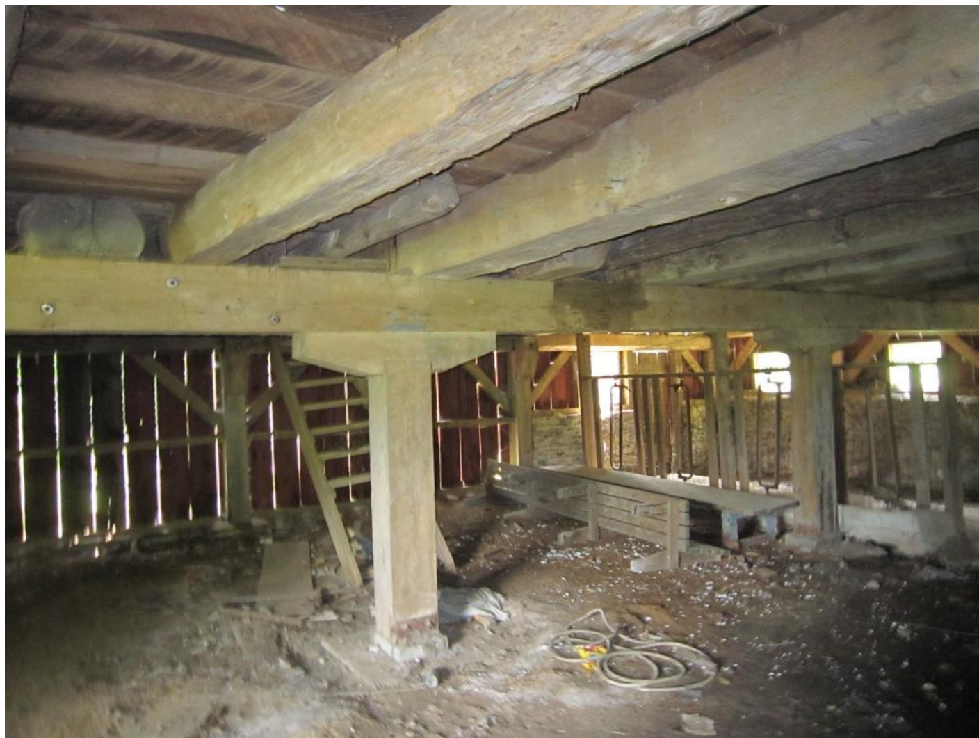
Figure 22. Interior of lower stable level, looking southeast. Ladder to upper level in center background, and 20 th century milking stanchions in right background.
