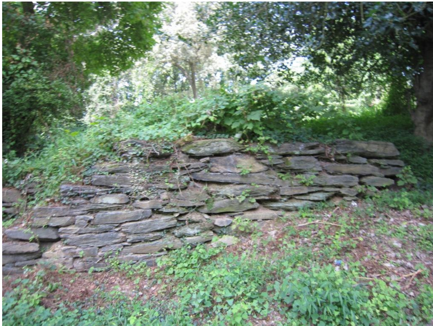
Figure 24. Dry stack stone retaining wall for banking earth.
