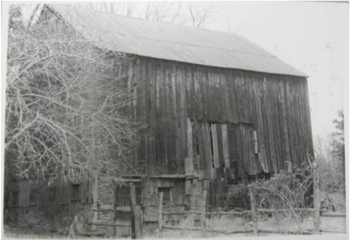
Figure 11. Stubbs Barn prior to renovations in the late 1980s. A note on the back of this photo, believed to have been written by John Armstrong, states: "Barn siding was always loose fitting. Tobacco barns were built that way. I was always told that the farm had originally been a tobacco [farm] long ago." Although tobacco was originally grown at "Shawfield," by 1850 the Stubbs family had switched to grain and corn cultivation, and this barn likely served those purposes. Courtesy: M-NCPPC
