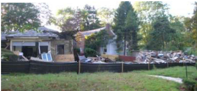
Left: Construction demolition debris from a single story dwelling unit.
