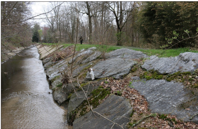
Figure C.8: Interim Stream Bank Repair without Concrete
