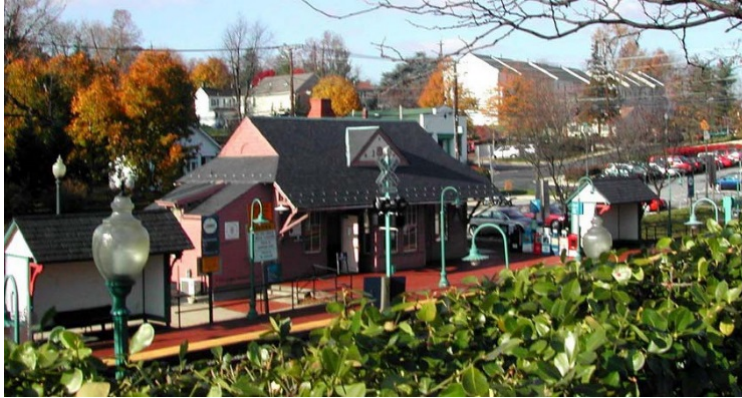
Germantown MARC Station
