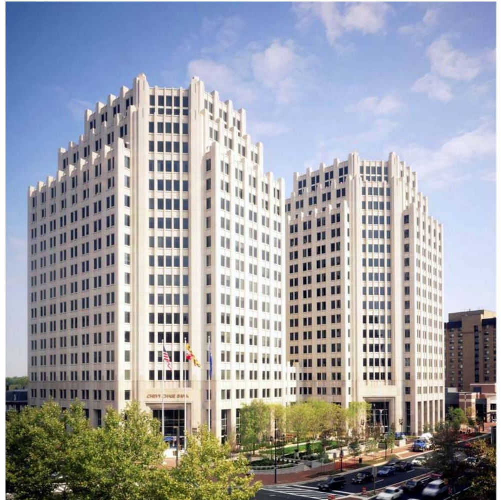
Chevy Chase Bank Building
