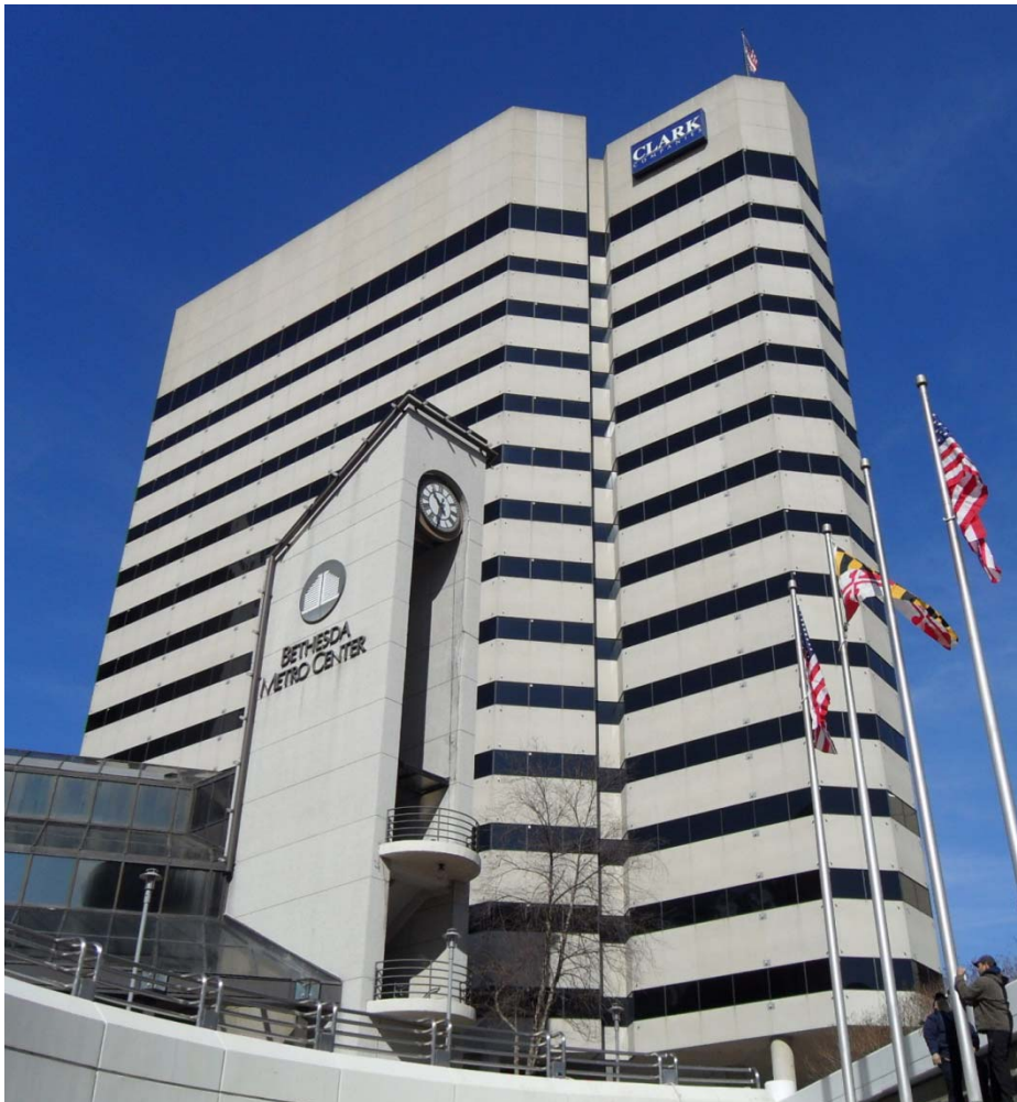
The Clark Building
