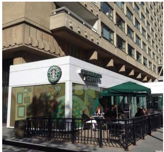
Liner building to retrofit existing structure and activate streetscape
