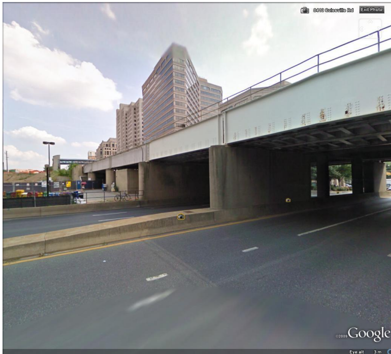
Figure 13 – Photo Looking Southeast as MARC / Metrorail Cross Colesville Road
