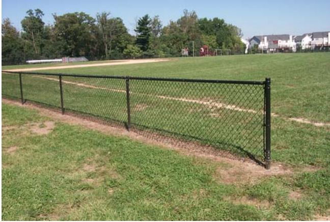
Figure 3.1.13.F. – Black Vinyl Coated Chain Link Fence with Top Rail
