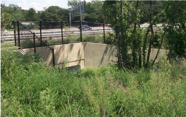
Figure 4.1.1.F–Chain Link Railing at Outfall Structure
