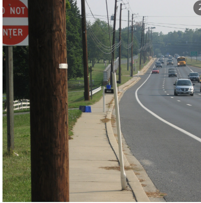
New Hampshire Avenue/Orchard Way north view
