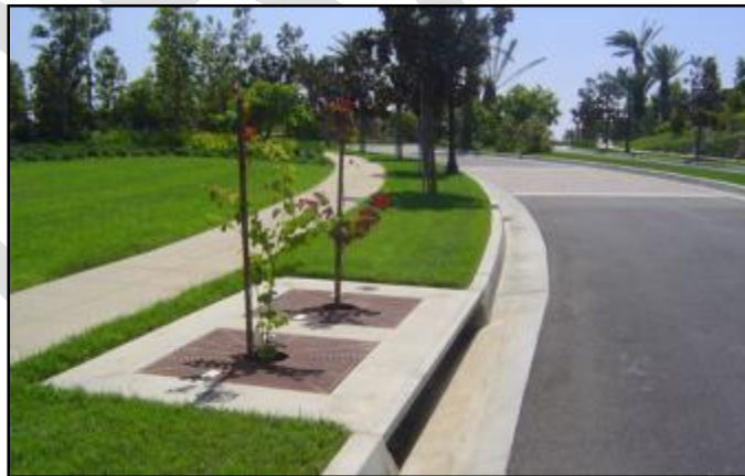
Figure 11: Examples of Filterra Inlets
