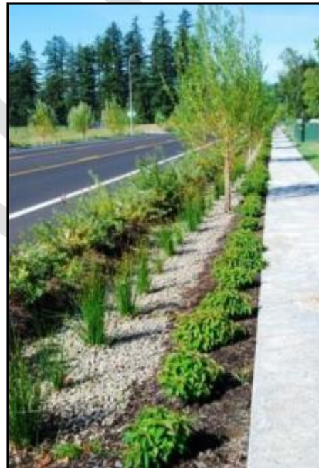
Figure 3: Example of Bio-swale
