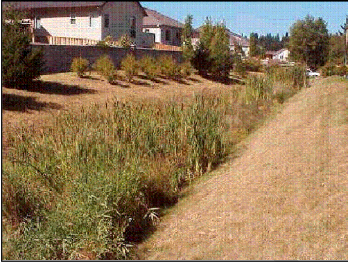
Figure 5: Example of Wet Swale
