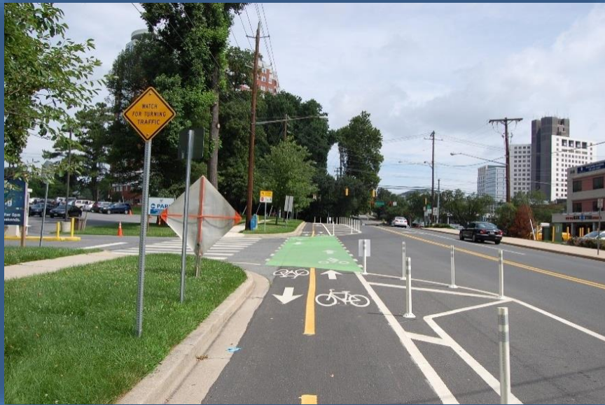
Separated Bike Lane on Woodglen Drive
