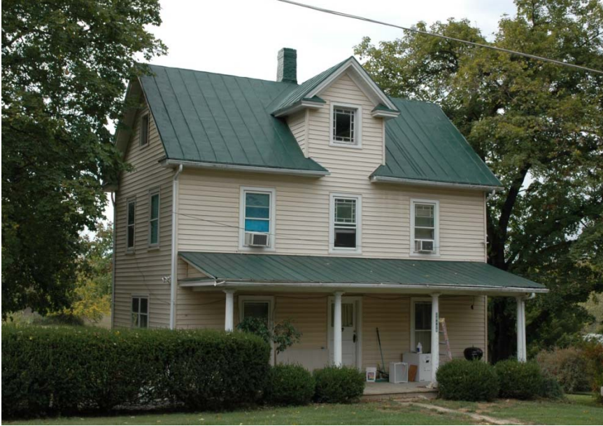
15/8-4 Lewis Easton House, 28408 Kemptown Road (c1895-1900)
