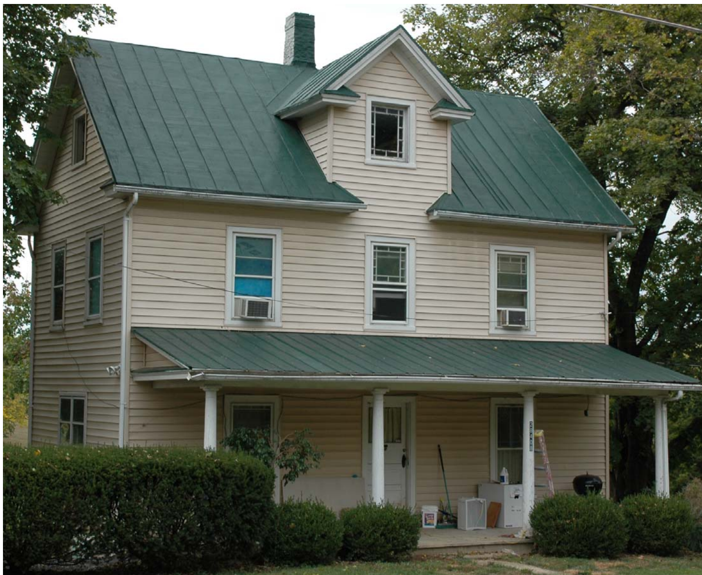
28418 Kemptown Road, North (front) façade, 11-1-2007
