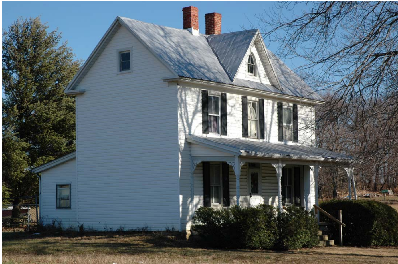
Front and west facades 28515 Kemptown Road, 11-2007
