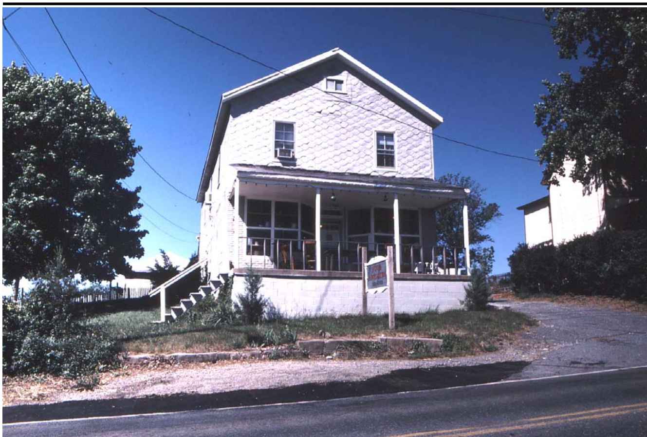
Harvey W Moxley Store (c1908-15), with side elevation of Harvey Moxley residence at right 28314 Kemptown Road, 1986 view (slide scan)
