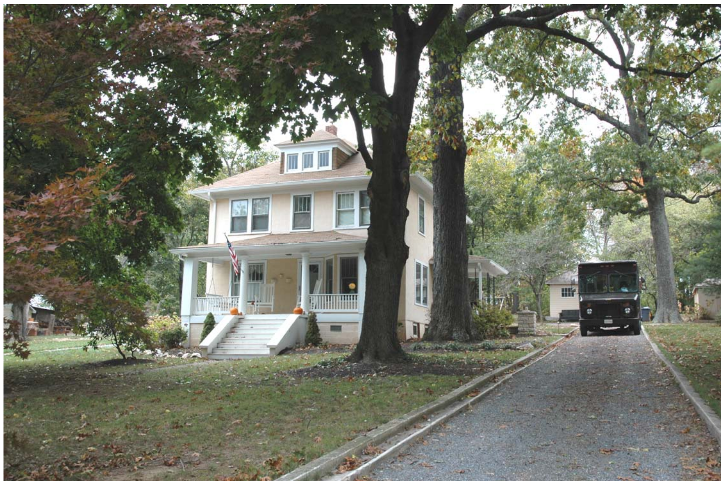
Ottie & Tressie Moxley House, 28411 Kempton Road View from Kempton Road, looking north, 11-2007
