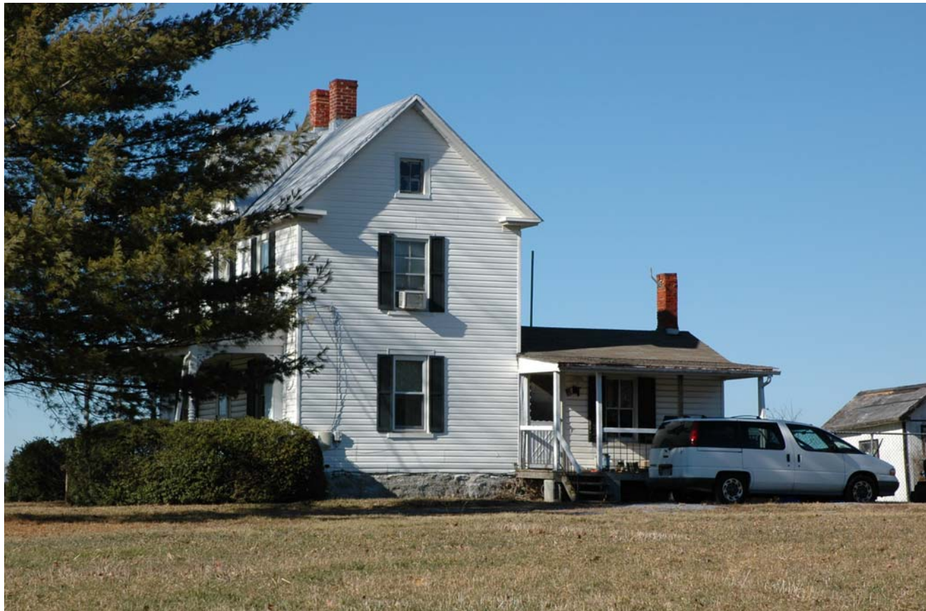
Front façade (left) and east façade with rear ell 28515 Kemptown Road, 11-2007
