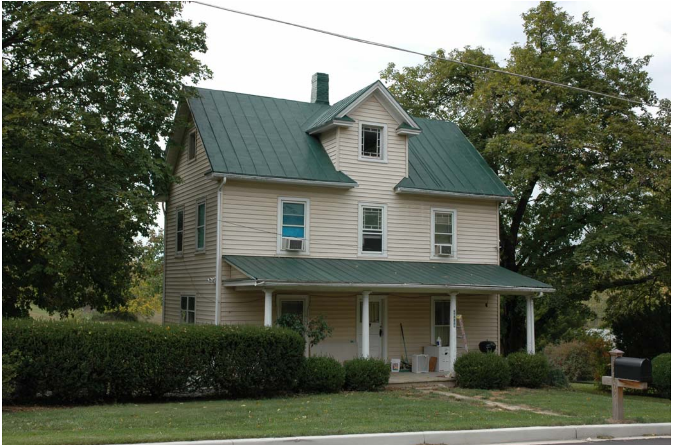
28418 Kemptown Road, View south from Kemptown Road, North façade, 11-1-2007
