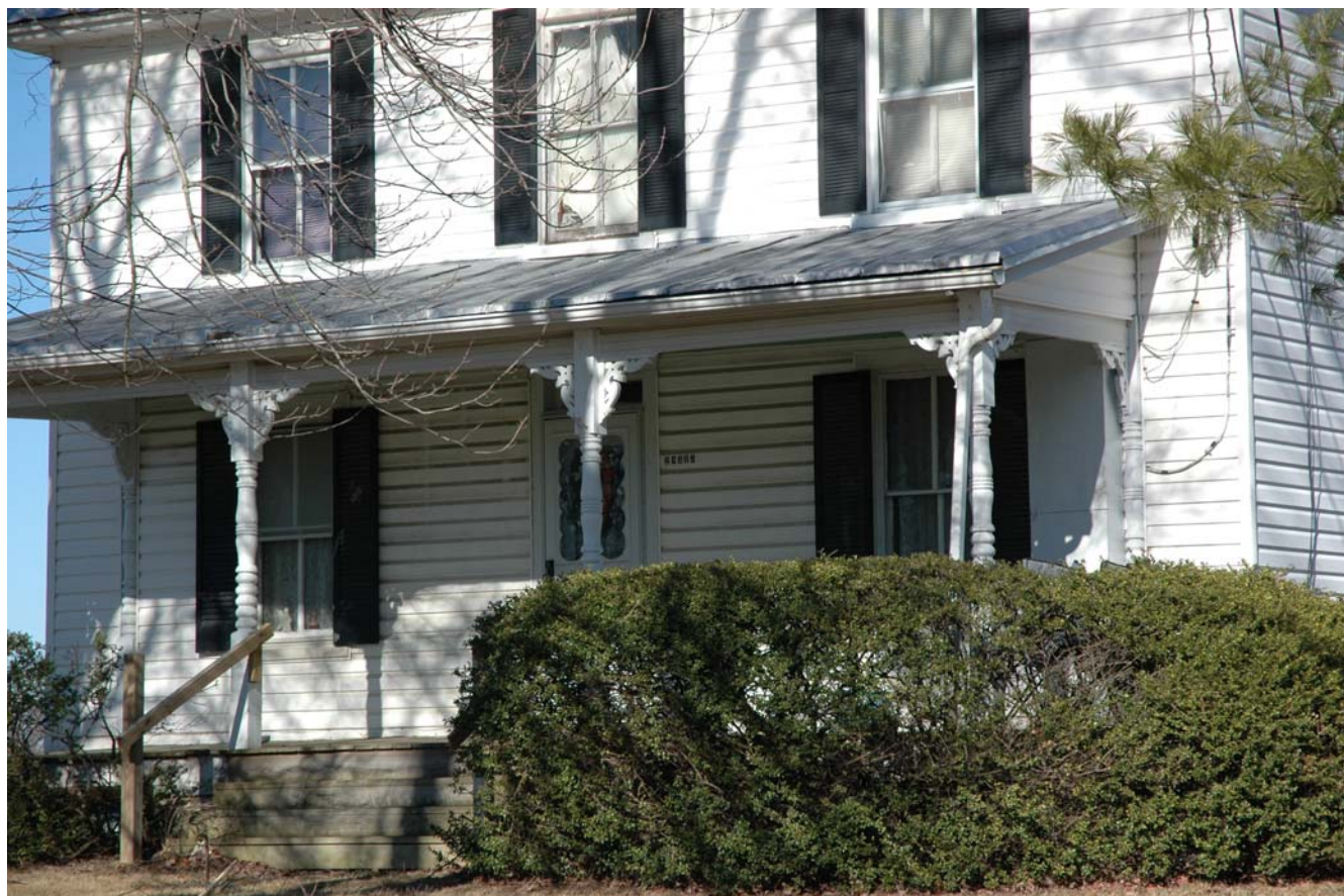
Detail, front facade 28515 Kemptown Road, 11-2007
