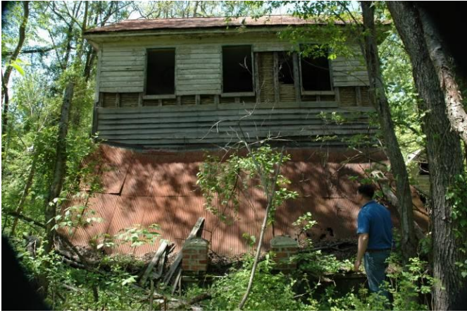
Front façade of double-door house with collapsed front porch, Site 2
