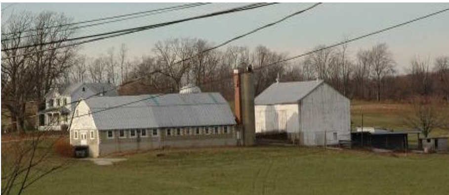
Dairy barn, silos, bank barn, Basil Warfield Farm (15/73)
