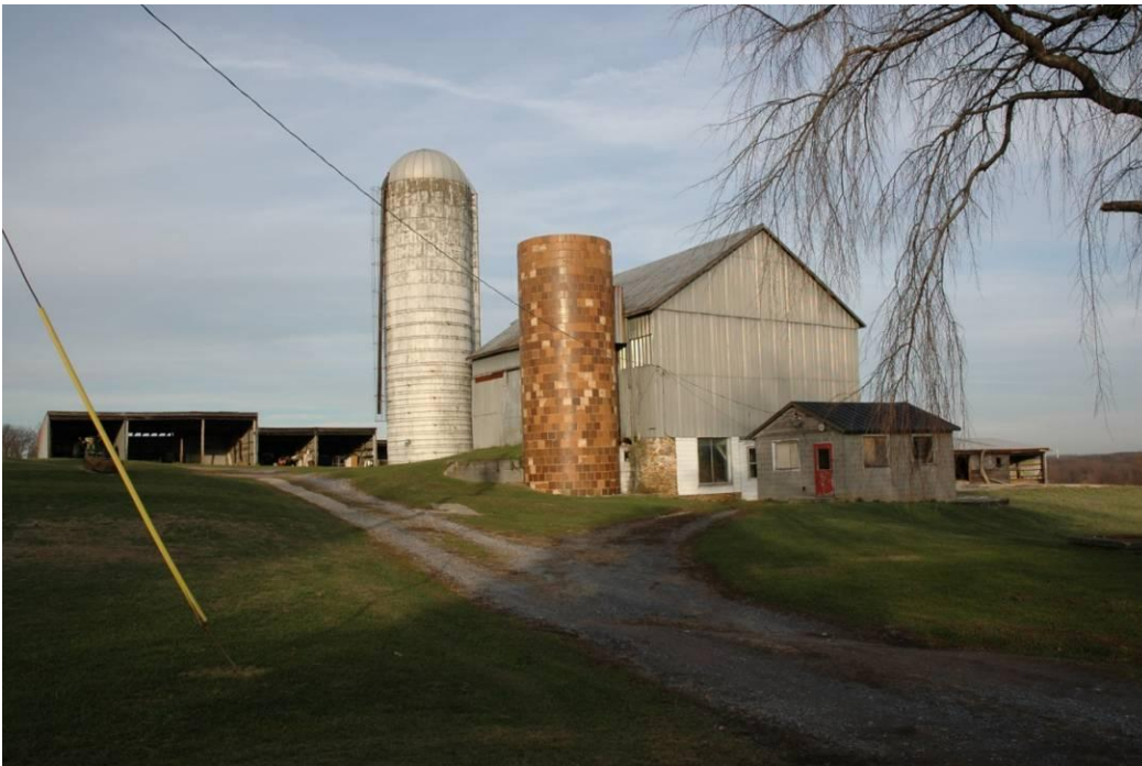
Bank Barn, Silos
