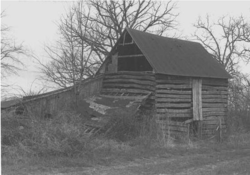
Barn on original Halterman Road site, 1979 view
