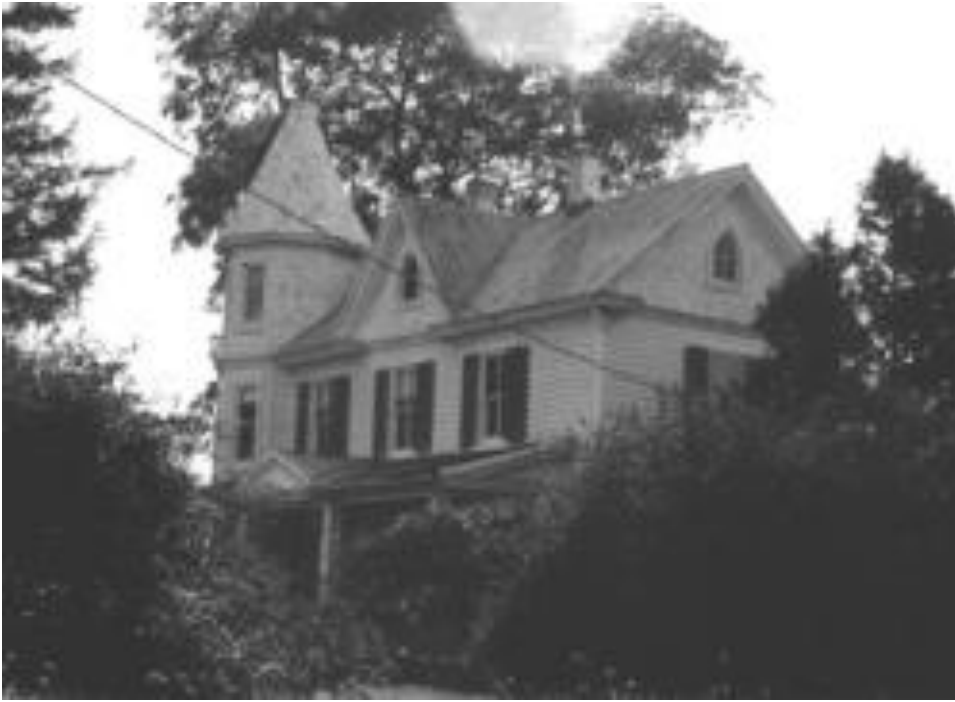
15/8 Clagettsville Historic District, Robert B. and Susan Moxley House, 28322 Kemptown Road with Queen Anne-influenced tower and wood-shingled siding
