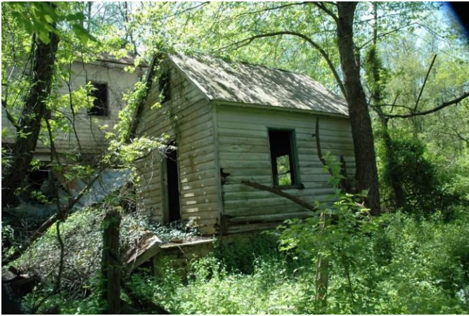
Summer Kitchen, Site 2
