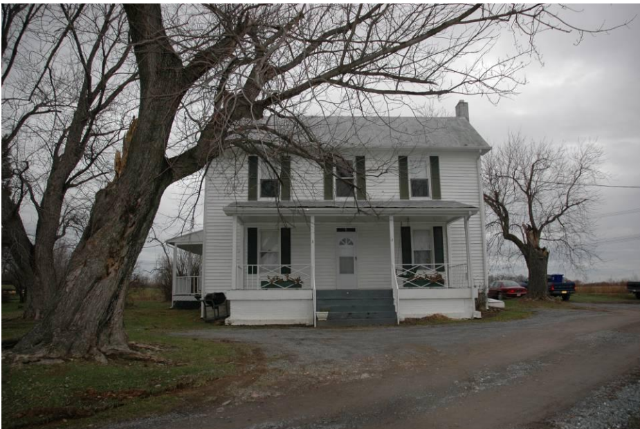
15/13 Shipley-Mullinix House, 27001 Long Corner Road
