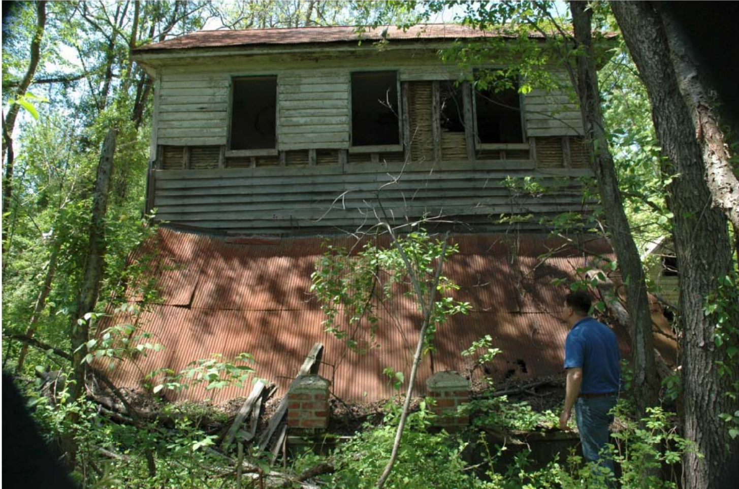
Wilson Warfield Site 2, Dual Entrance House, May 2008
