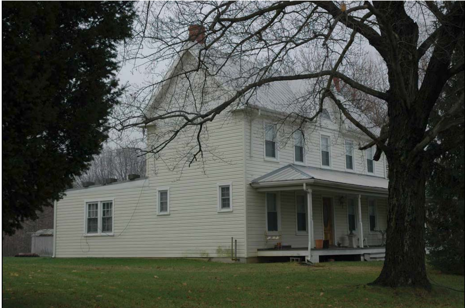
Dwelling House, Front and Side Façades, December 2007
