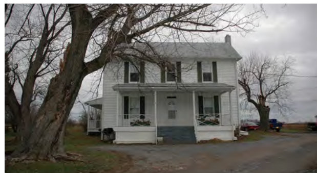
15/13 Shipley-Mullinix House, 27001 Long Corner Road
