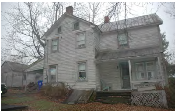
Dwelling House, southern façade, facing Mullinix Mill Road
