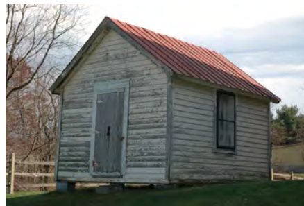
Domestic outbuilding, demolished October 2010
