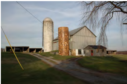
Bank barn, silos
