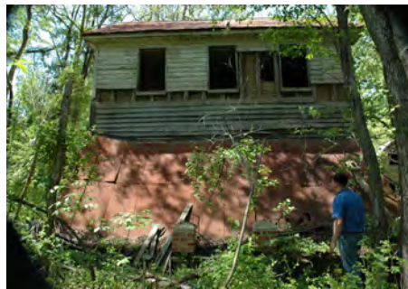
Front façade of two-door house with collapsed front porch, Site 2
