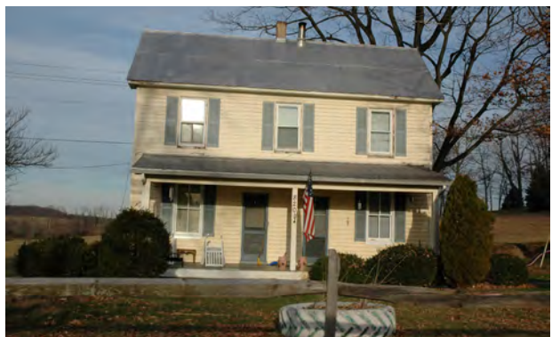
15/73 Basil Warfield Tenant House, 8201 Damascus Road
