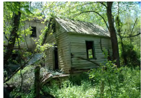
Summer kitchen, Site 2
