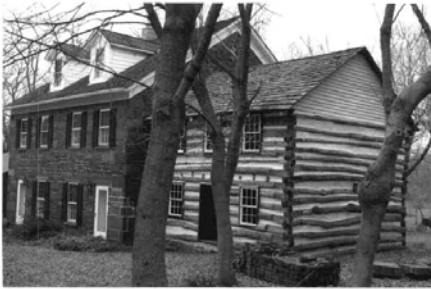
Barn moved to Quarry Master's House, 19816 River Road
