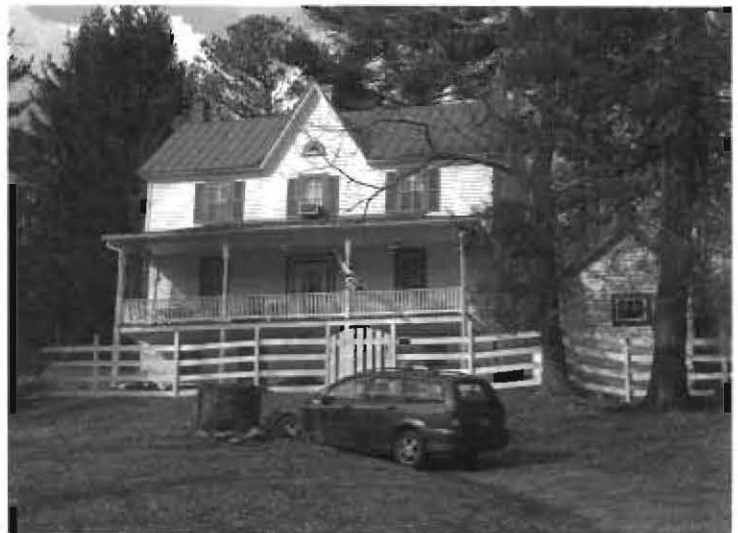
15/71 Chrobot House (Margaret Price House), 24724 Hipsley Mill Road, with Germanic influence—banked into a hillside with a two-story front porch and basement kitchen
