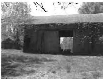
Barrack barn, Site 1
