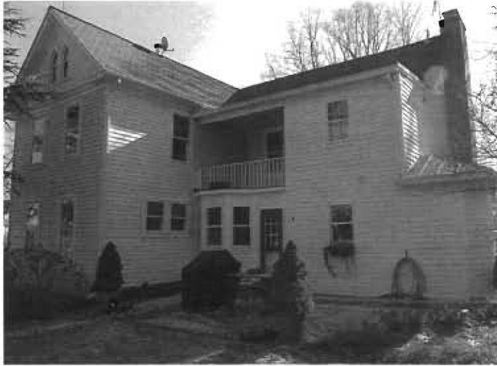
15/5 Molesworth-Burdette House, 28600 Ridge Road, with two-story rear porch (now partially enclosed)
