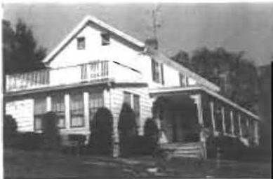
Log house, no longer standing
