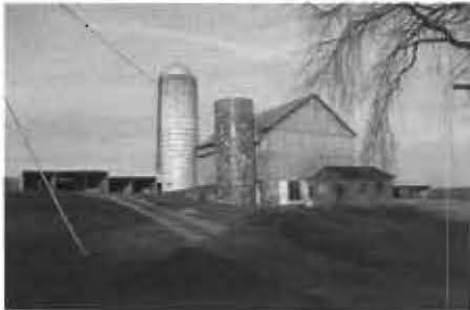
Bank barn, silos
