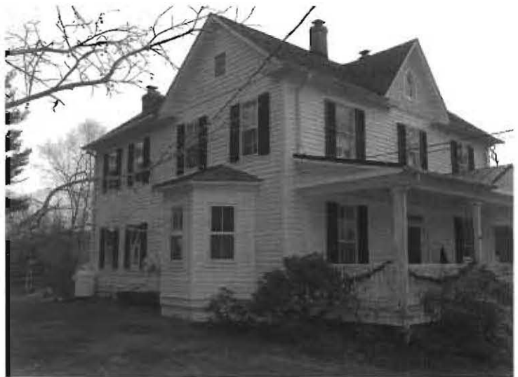
15/17 Sarah Brandenburg House, 26301 Mullinix Mill Road, with rear ell, Queen Anne-influenced shingles, gables, and bay windows
