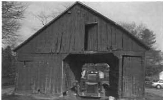
Combination corn crib-granary (granary on left)
