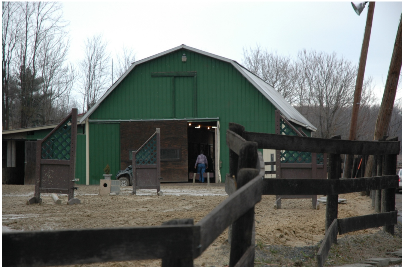
15-4 Alfred Baker House Barn: southwest and southeast façades. Sandra Youla, 2.6.2008
