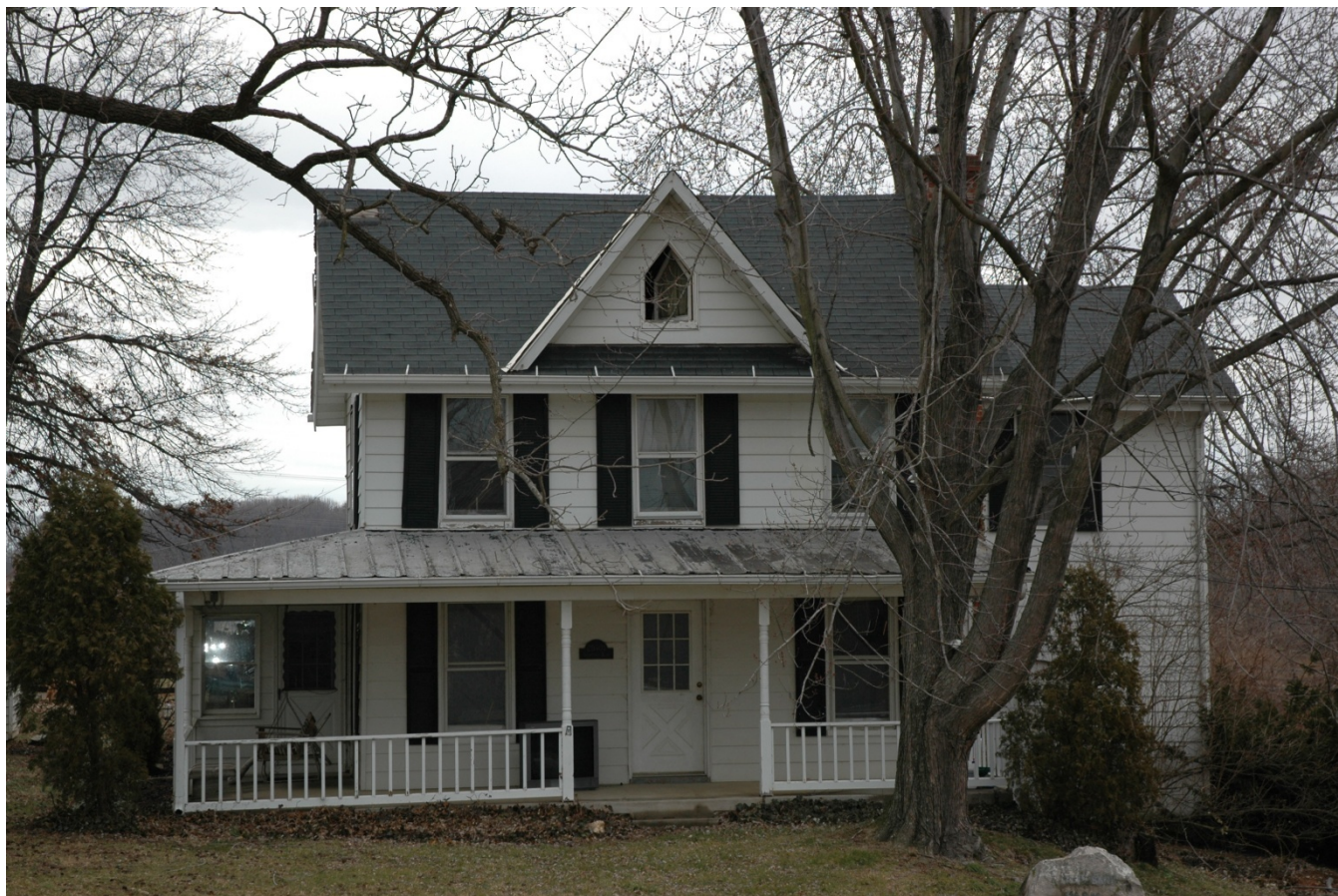
15-4 Alfred Baker House Dwelling House: southwest façade. Sandra Youla, 2.6.2008
