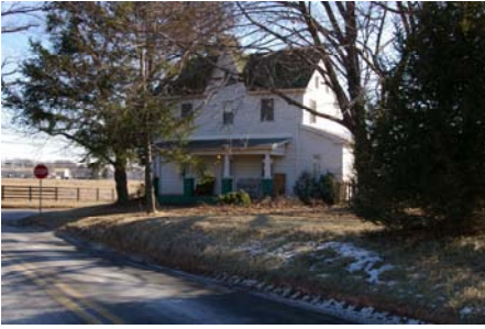
Franklin & Grace Allnut House, c1920, 6760 Hipsley Mill Rd
