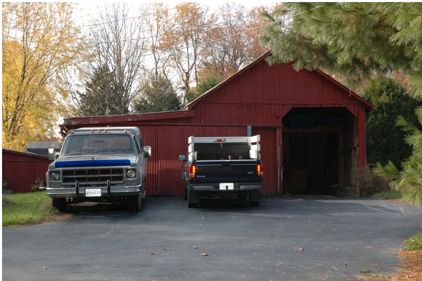
Walter and Ida Allnut House, 6920 Damascus Road Garage with shed extension, 11-2007
