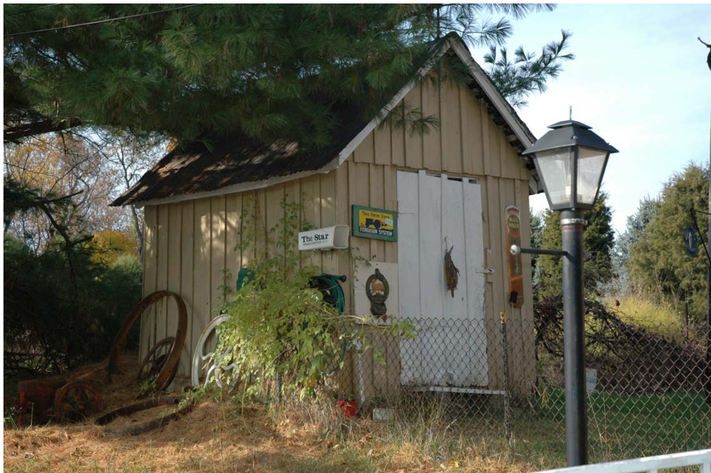
Outbuilding, possible smokehouse, 11-2007
