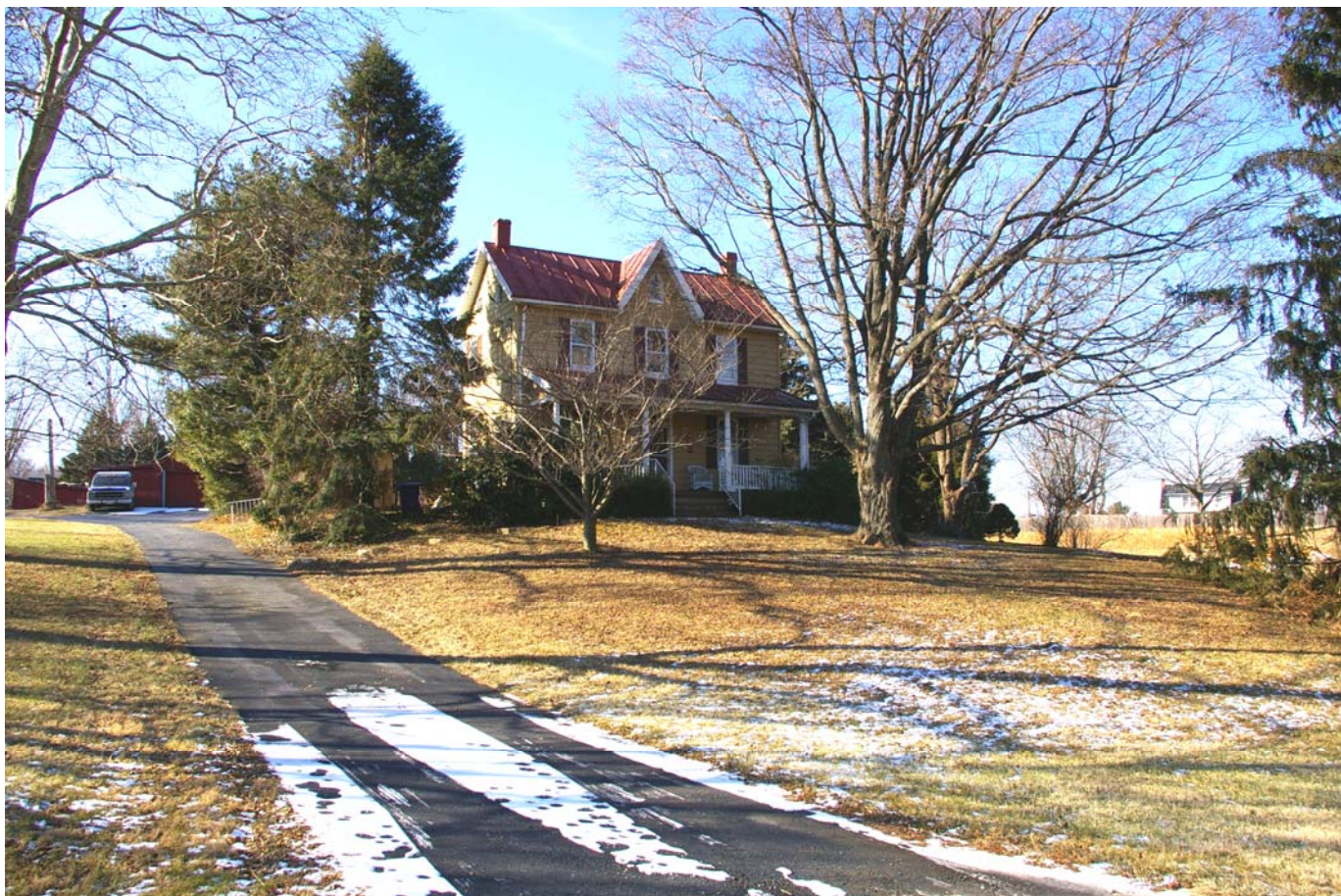
Walter and Ida Allnutt House, 6920 Damascus Road Overall view south from Damascus Road, 1-2009
