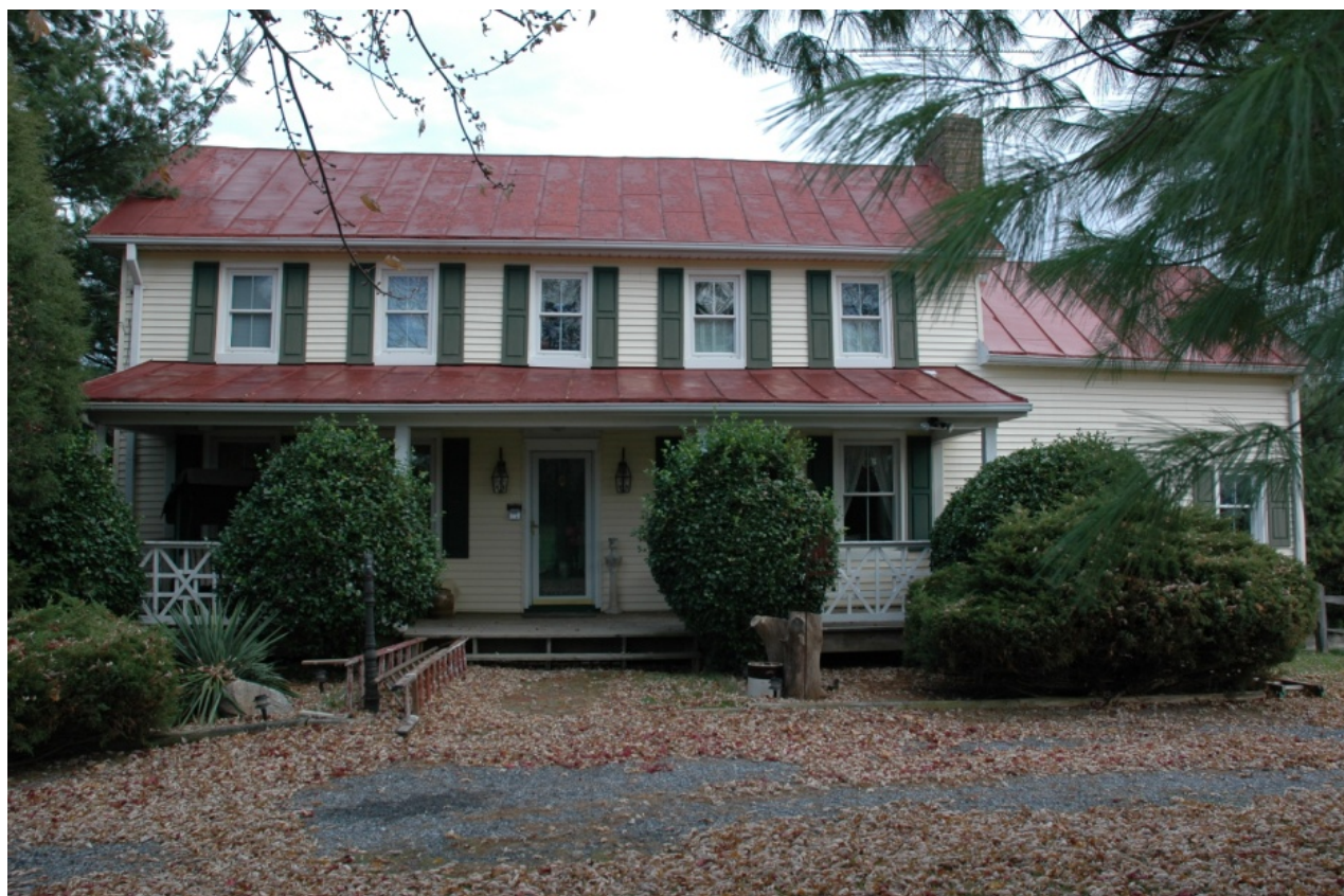
Luther Moore Farm, Dwelling House Main (south) façade 11-2007
