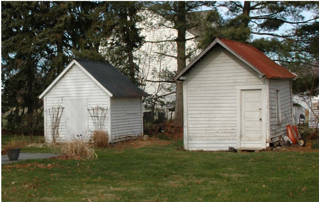
#15-17 Brandenburg Farm, Domestic Outbuildings including a Smoke House (left) and Summer Kitchen (right), with house on neighboring property behind, Sandra Youla, 12.18.2007 Carriage House (ca. 1870 to
