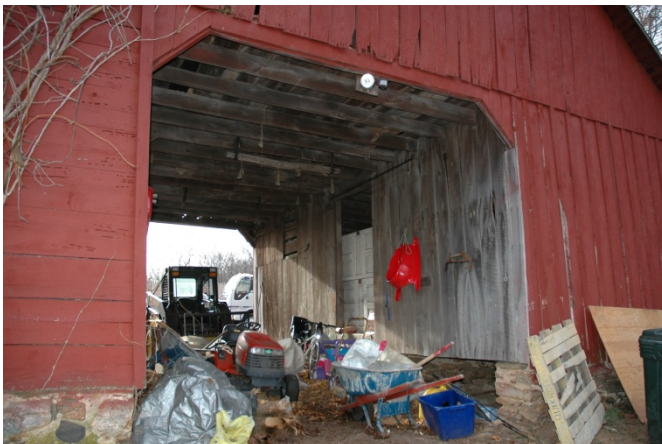
#15-17 Brandenburg Farm, Corn Crib and Granary, Northeast Façade and Interior Wall of Granary, with tight vertical boards, Sandra Youla, 12.18.2007
