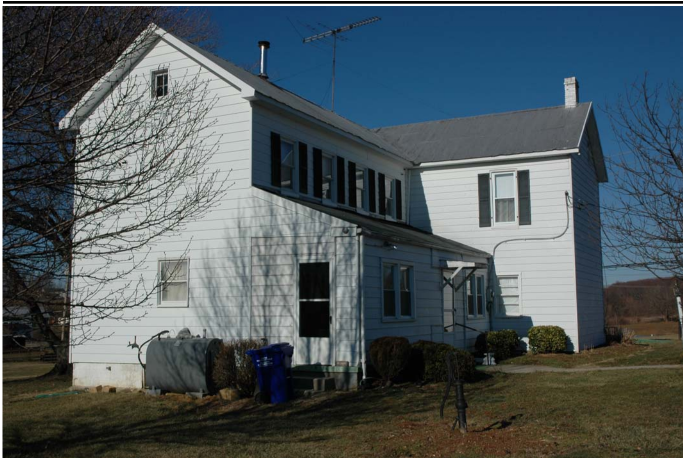
John Moxley House South (rear) facade, left, and east façade, right. 1-2008
