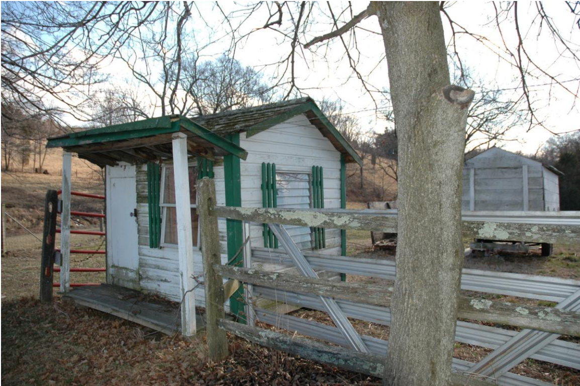
Dairy House: Northeast and northwest facades, looking southwest.
