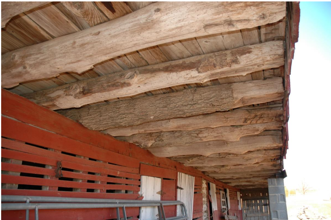
Bank Barn: Southeast Façade, underside of projecting forebay.
