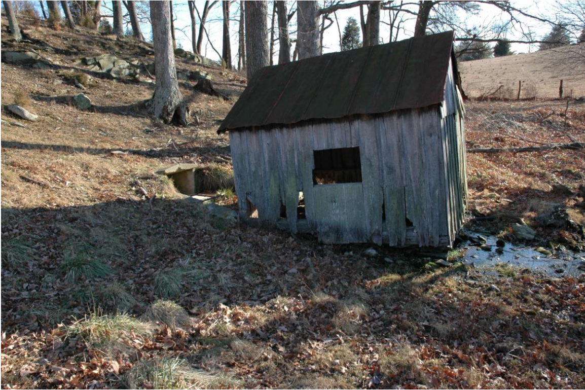
Spring House: Northeast façade, looking west.
