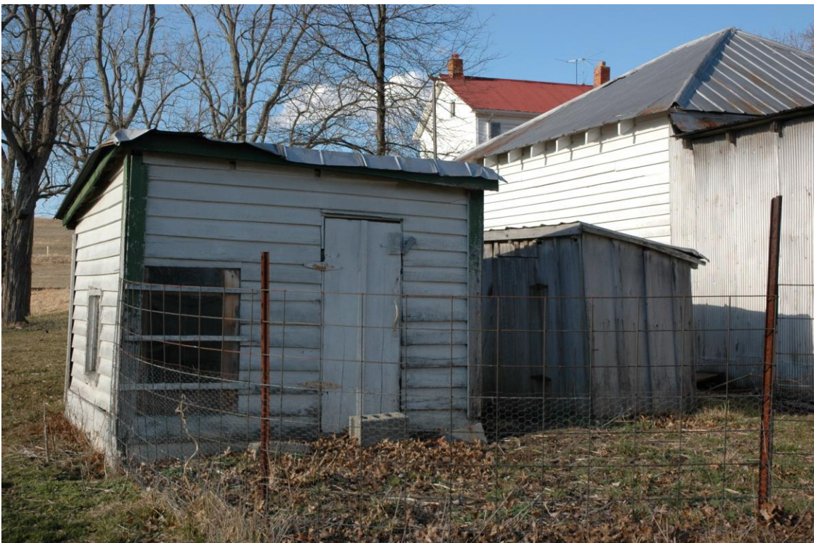
Two Outbuildings, function unknown: Southeast facades, looking northwest.
