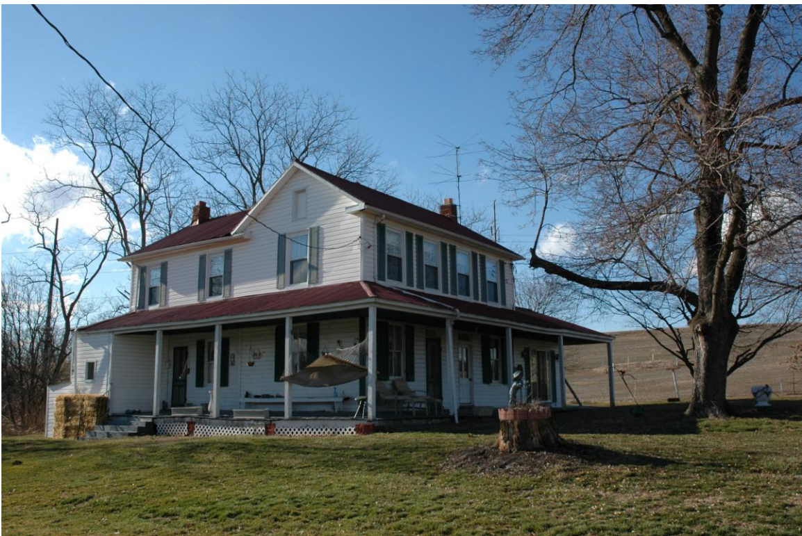
Dwelling house: southwest and southeast facades, looking north.
