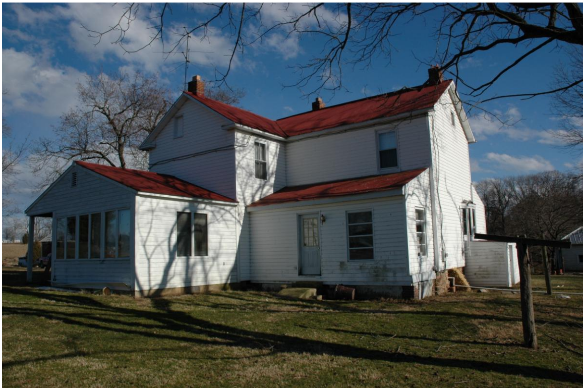
Dwelling House: Northwest and southwest facades.
