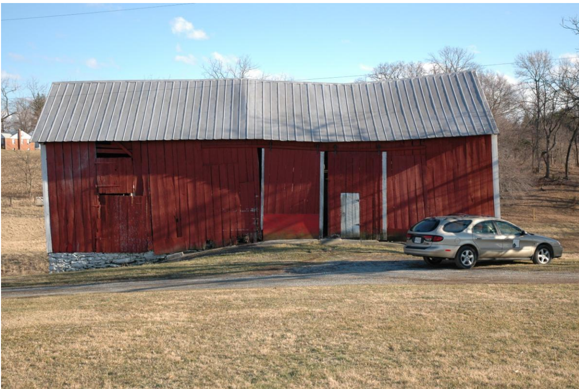
Bank Barn: Northwest façade, looking southeast.
