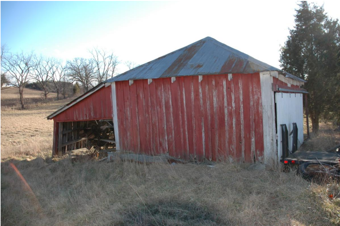
Vehicle and Equipment Storage Shed: Northeast façade, looking southwest.
