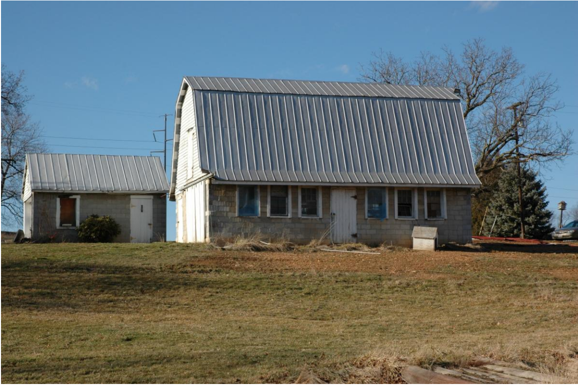
Milk House and Dairy House: Southeast facades, looking northwest.
