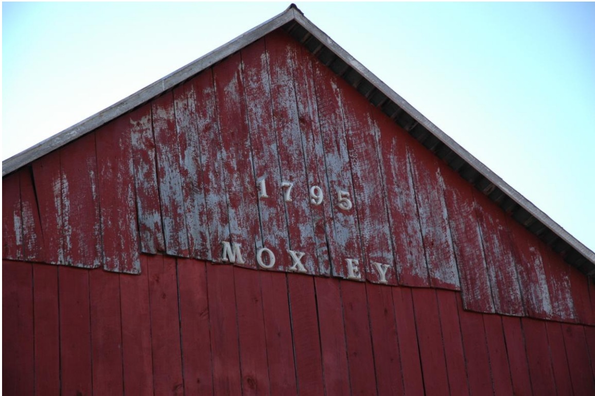
Bank Barn: Northeast gable.
