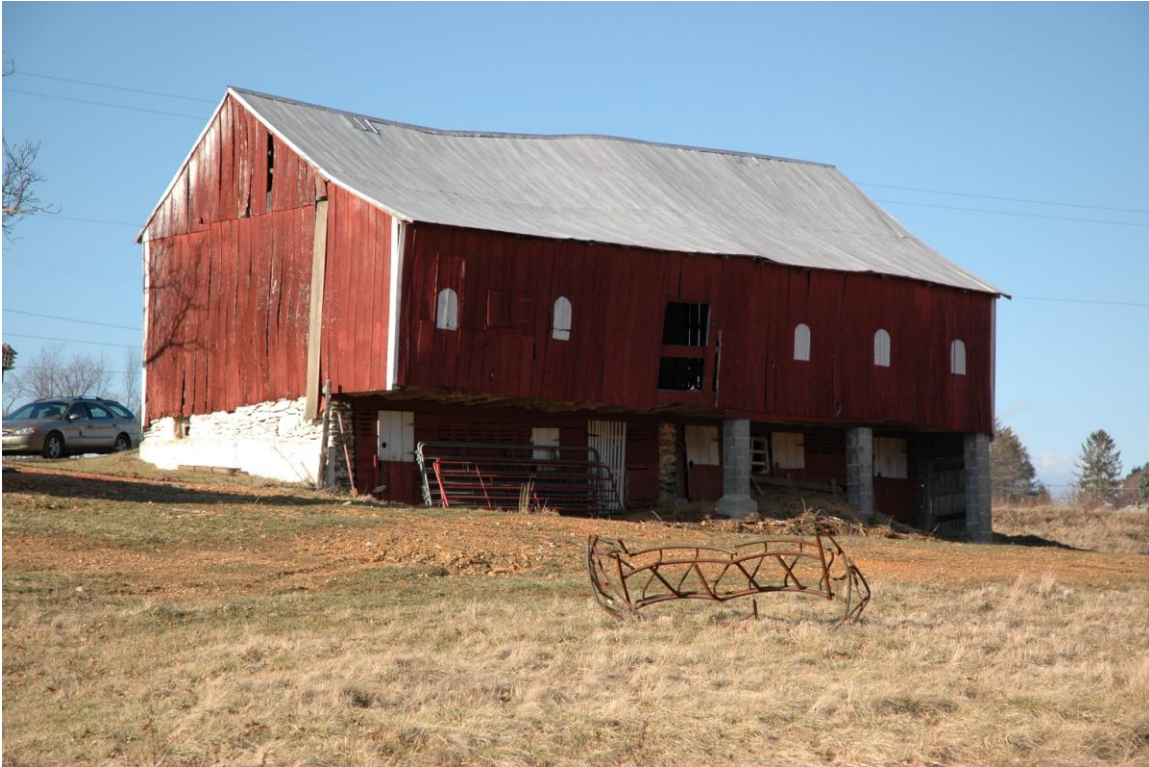
Bank Barn: Southwest and southeast facades, looking north.
