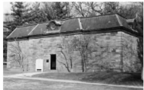
Washington Aqueduct Control Gate House (1850s)
