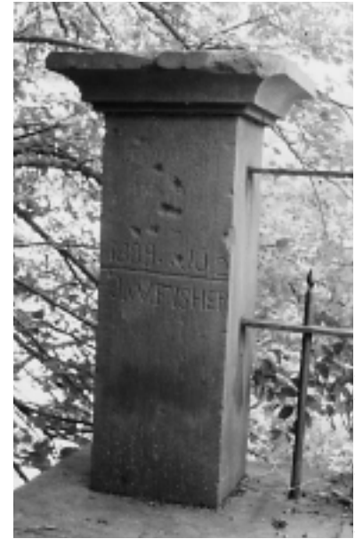
Seneca Aqueduct, detail (1831)
