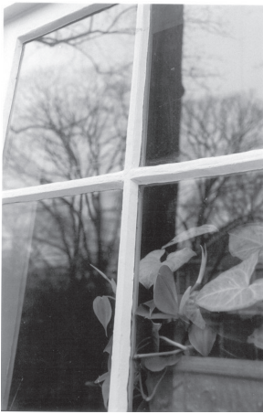
Restoring old windows qualifies for tax credits. 7113 Holly Ave., Takoma Park.
