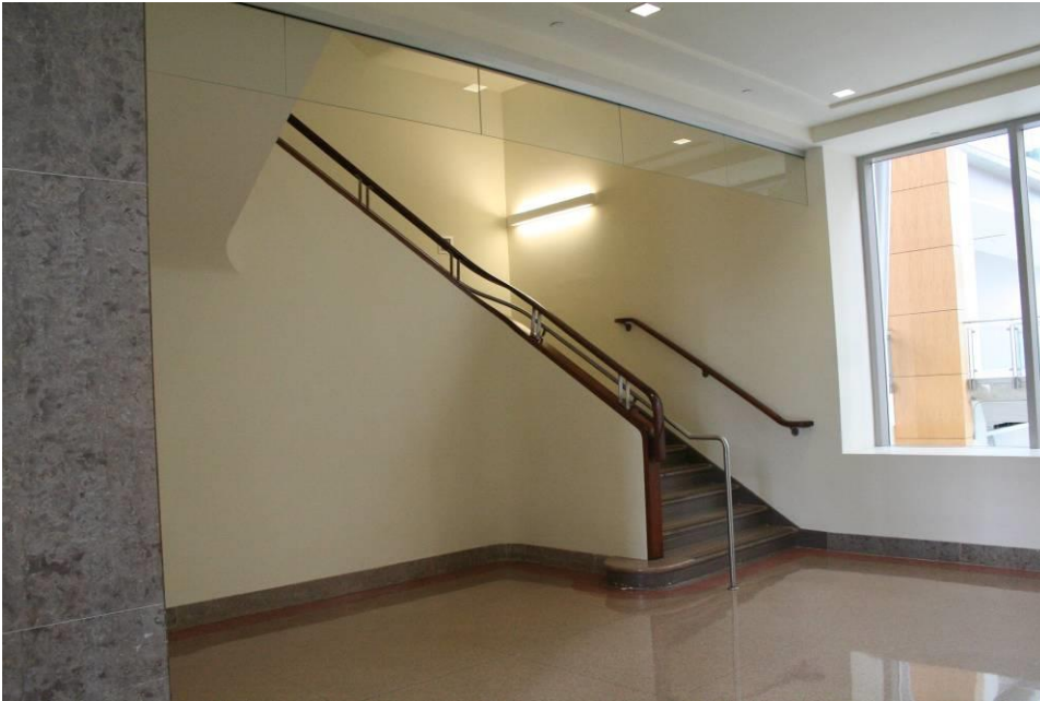
Stairwell with added railing (for code purposes), rear public stairwell lobby, 2011
