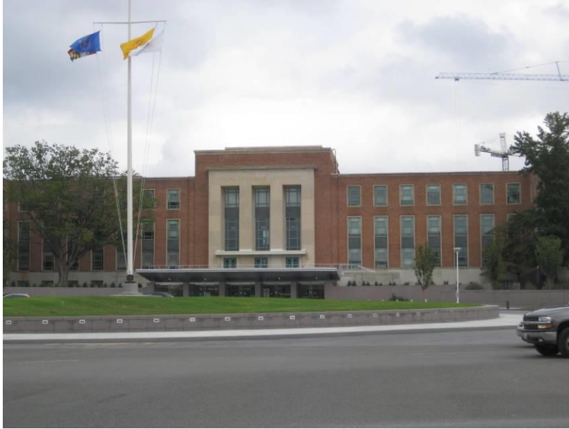
Front façade, partial view, with flagpole and partially submerged new entry, 2011
