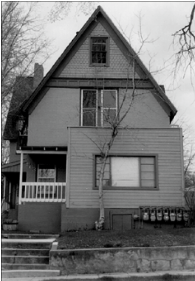
Guideline 18.4: Design a new addition such that the original character can be clearly seen. This addition to the front of a historic house is inappropriate. (Salt Lake City, UT)
