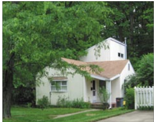
Guideline 18.7: Eave lines on the addition should be lower than those of the historic building.
