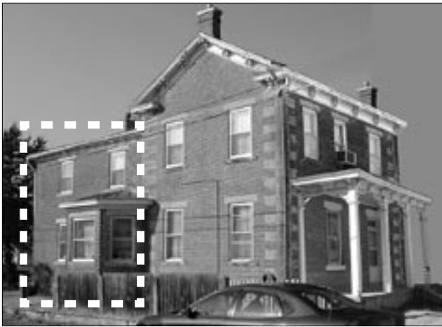
Guideline 17.1: Preserve an older addition that has achieved historic significance in its own right. This addition, for example, should be preserved. (St. Genevieve, MO)
