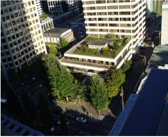
Benefits of green roofs include reducing stormwater runoff and reducing energy use.
