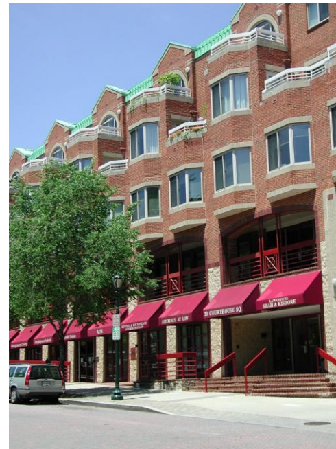
Residential building over ground floor retail, Rockville, Town Center
