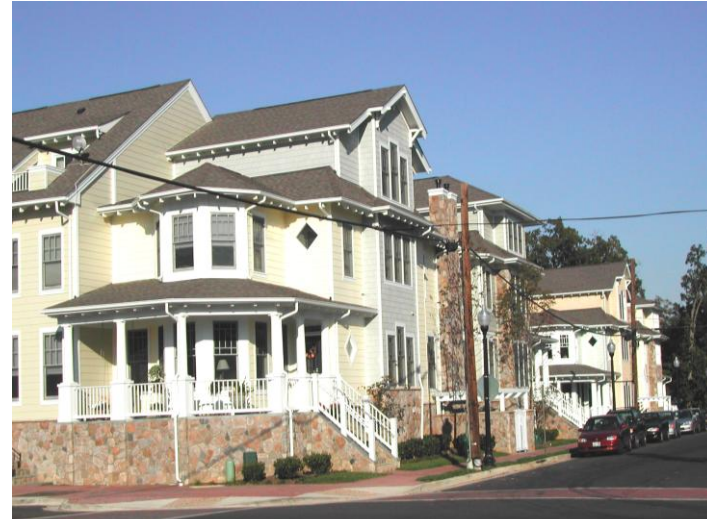
Varied roof lines on residential development, Clarendon, Virginia
