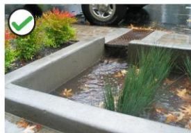
Allow stormwater to serve a purpose, such as watering plants, before entering the storm drains.
