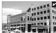
A part of this building is a parking structure that is set back from the front and sides of a retail wrap. The openings in the parking section reflect window proportions similar to those seen historically in the area.
