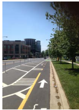
Woodglen Drive separated bike lane
