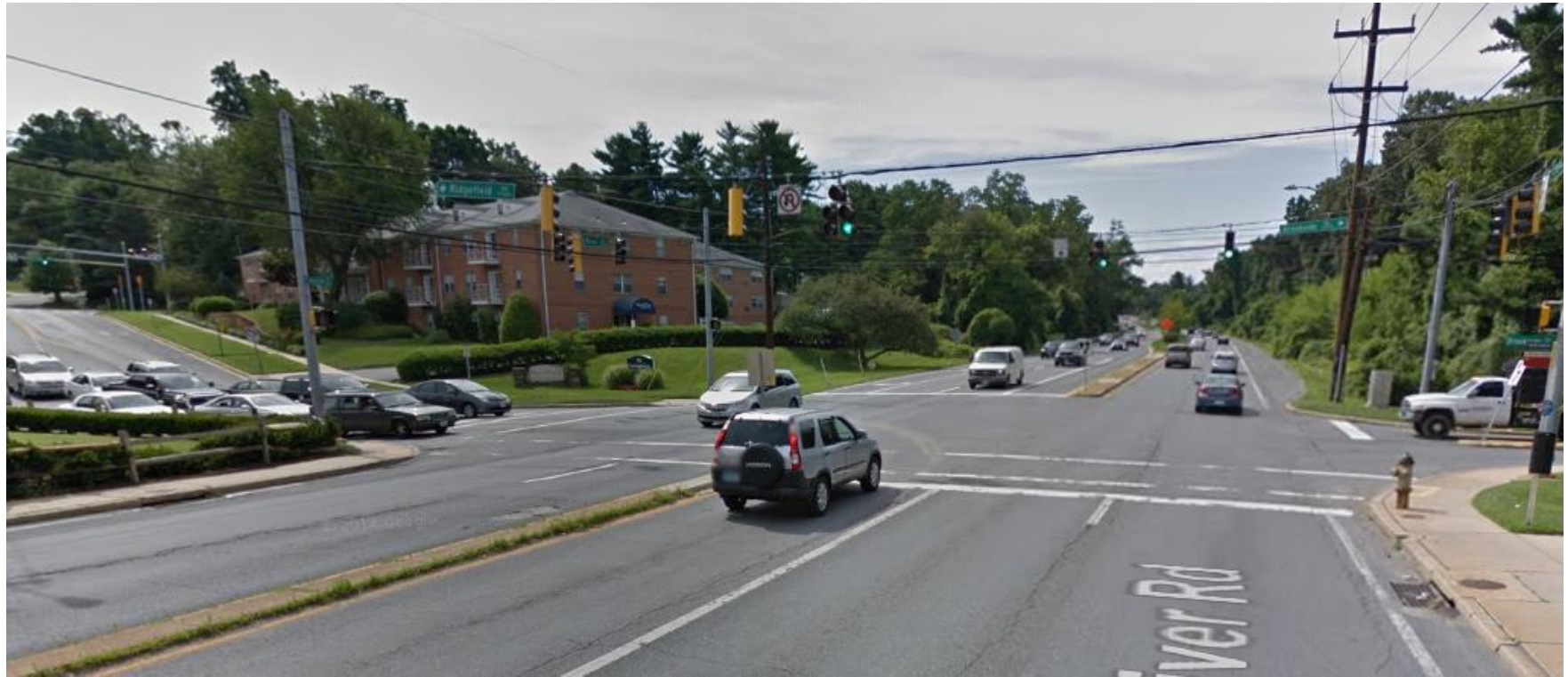
River Road at Ridgefield Road, looking westbound
