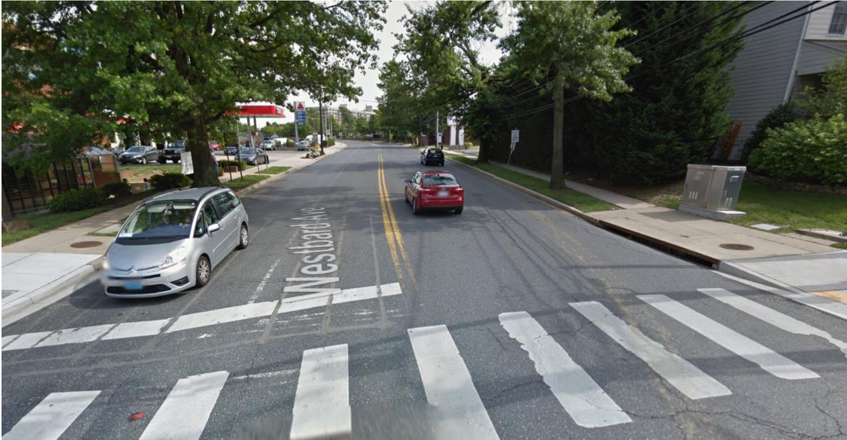
Westbard Avenue at Ridgefield, looking southbound
