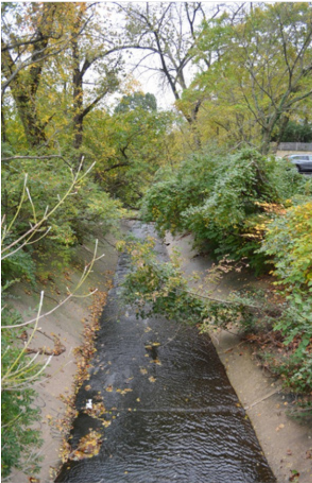
Willett Branch is contained in concrete channels
