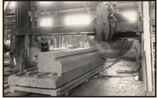
Large stone-cutting machine at Fuller Plant
