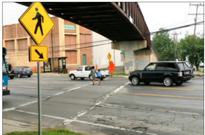
Pedestrian access across River Road is difficult
