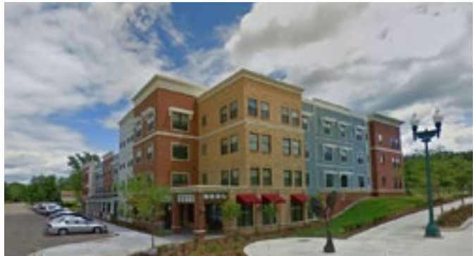
Affordable housing units over ground-floor retail
