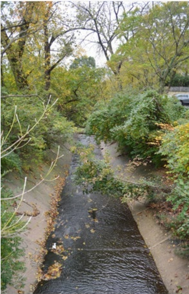
Willett Branch is contained in concrete channels
