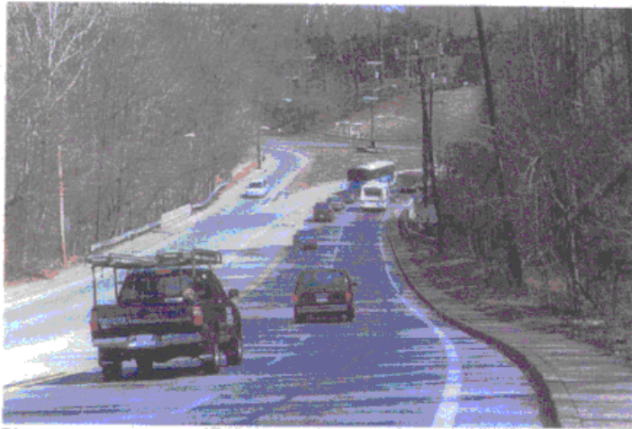
Piney Branch Road at the Bridge over the Northwest Branch
