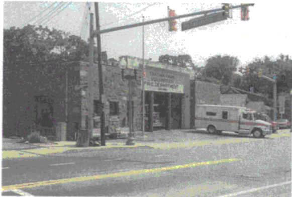
Reconstruct the Takoma Park Fire Station
