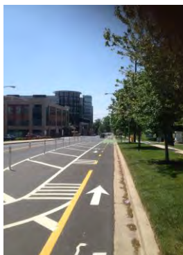
Woodglen Drive separated bike lane
